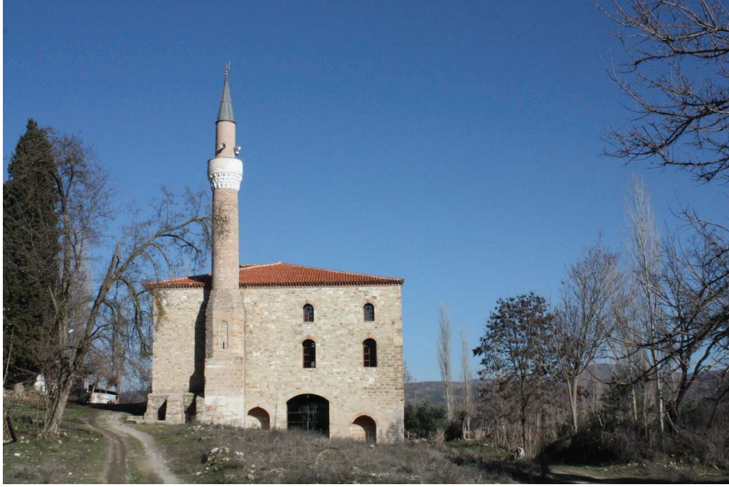
Figure 3.27. View of Pazaryeri Mosque and the surrounding site from the west. (Source: Büyükkılıç-Koşun 2018)
