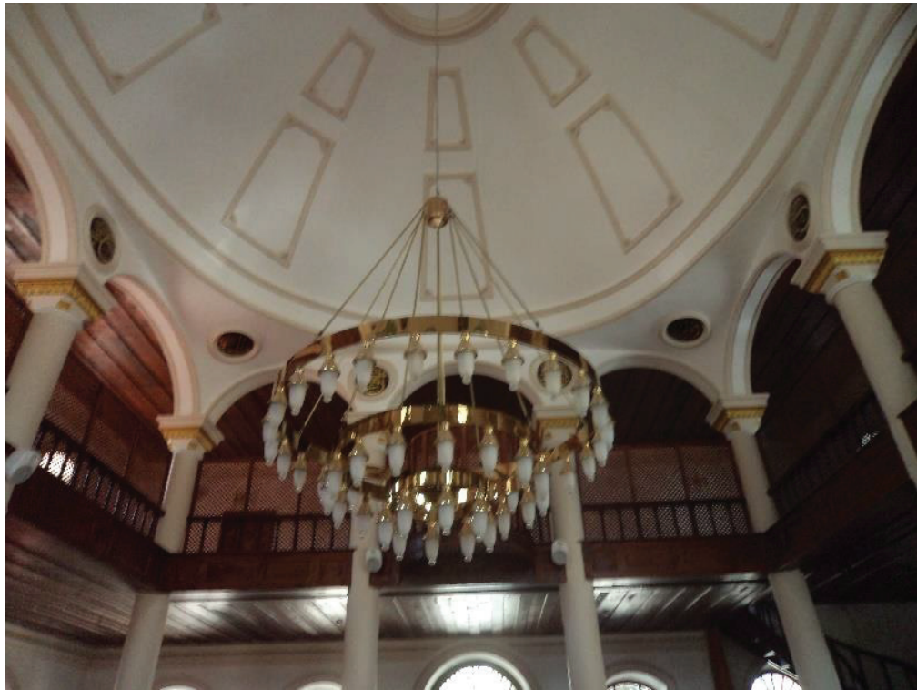
Figure 3.40. Timber columns, arches, dome of Çarşı Mosque.
