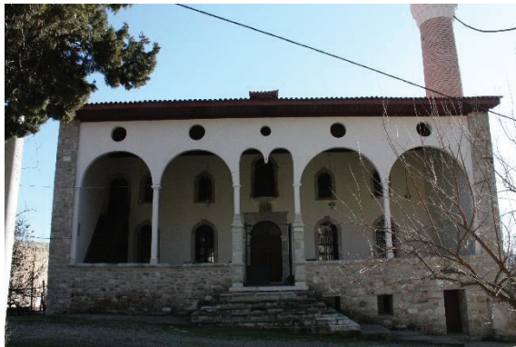
Figure 3.28. View of Pazaryeri Mosque's last comers' hall at its north.
