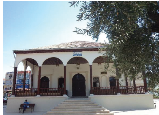
Figure 3.39. Çarşı Mosque as viewed from north.
