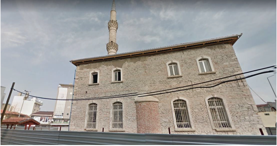
Figure 3.41. Construction technique of the wall, Çarşı Mosque. (Source: Google Maps 2015)
