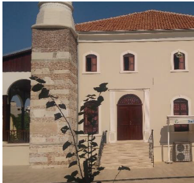
Figure 3.38. Çarşı Mosque as viewed from west.
