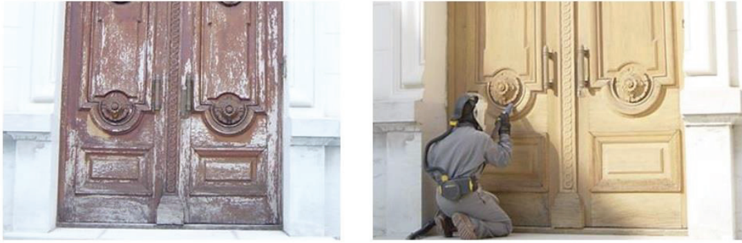
Figure 2.9. Cleaning of the surface of a historical door. (Source: Kesik et al. 2015, 1105)
