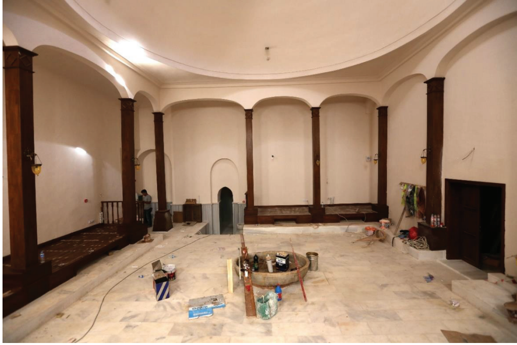
Figure 2.8. Renewal of columns in Bursa, Reyhanpaşa Bath. (Source: Bursa Municipality n.d.)
