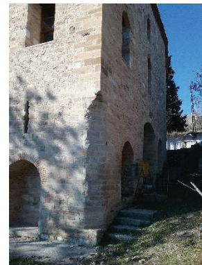
Figure 3.29. View of Pazaryeri Mosque's eastern façade.
