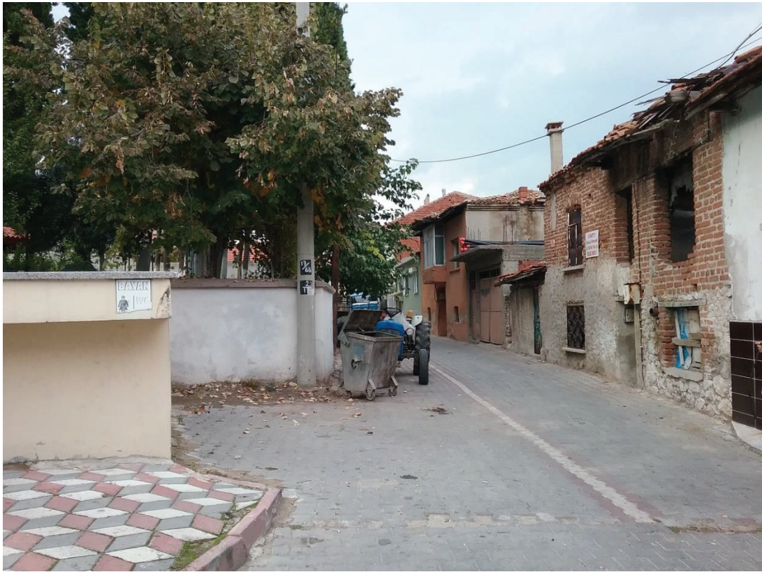
Figure 3.16. View of Kabasakal Mosque's courtyard wall's southeastern corner and wall of underground toilet in front of it, 79/B street and houses at the east.
