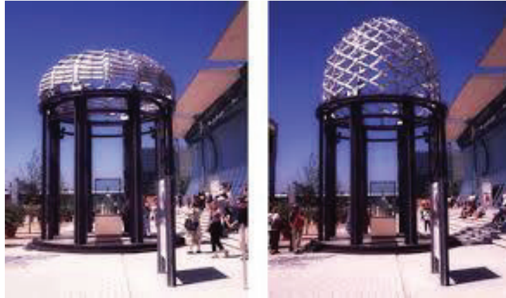
Figure 1.18. Open and Closed Form of Iris Dome (Source: Google Images, 2018)
