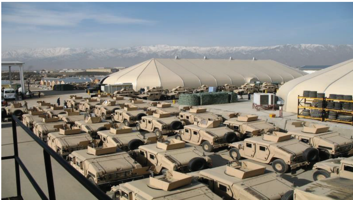
Figure 1.4. Rapidly Deployable engineered membrane structures (Source: © Sprung Instant Structures, 2018)
