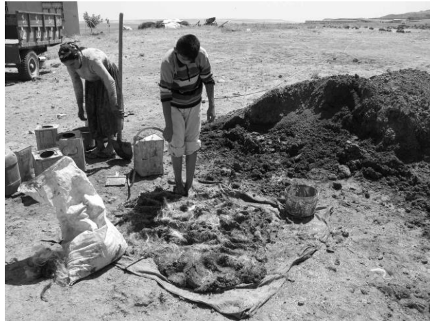
Figure 2.7. Boy helping his mother mix goat hair and salt into the clay soil and knead it with feet in Çarıklı Village, Diyarbakır. (Source: Parker, 2011)
