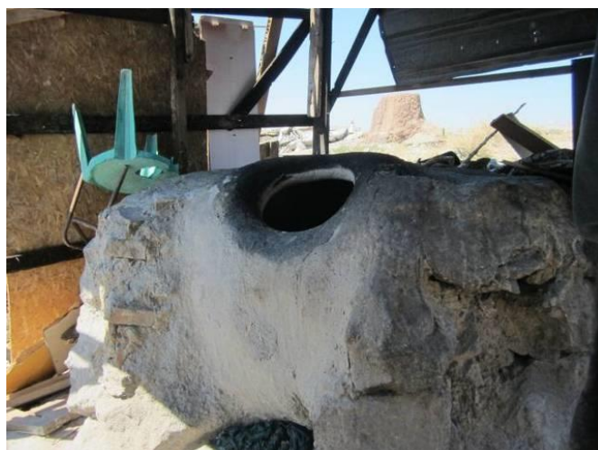
Figures 2.31. View of a tandır oven in Kadifekale. The tandır core is covered with concrete and rocks from the outside to increase the durability.
