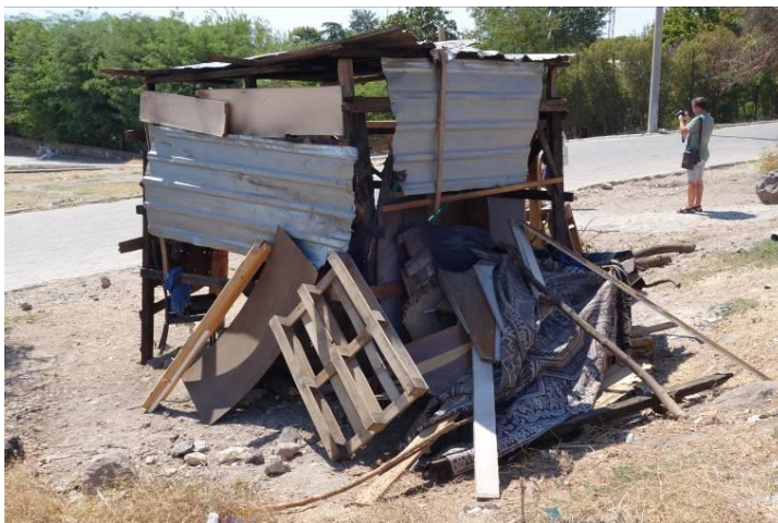
Figure 2.25. Different protective shelter adjustments. (Source: photos by Can Gündüz)
