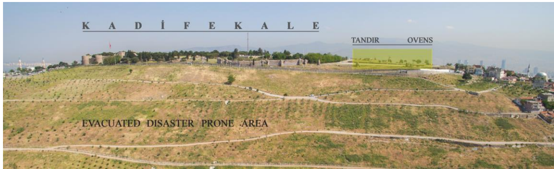
Figure 2.18. Location of the tandır ovens inside the citadels of Kadifekale, view from Buca. (Source: İzmir History Project Centre)
