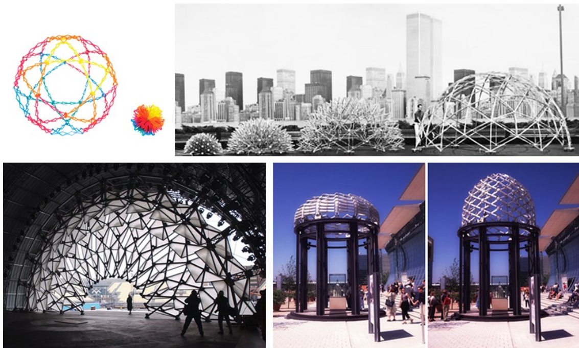
Figure 2.1.12. Hoberman Sphere (up left), Expanding Geodesic Dome (up right), Hoberman Arch (down left), open and closed Iris Dome (down right) (Source: Hoberman Assc. and Salt Lake Tribune webpages, 2017)
