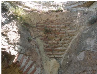
Figure 4.166. North East pendentive of the South West Halvet
