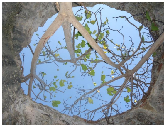
Figure 4.141. Dome plaster of Cleaning Cell
