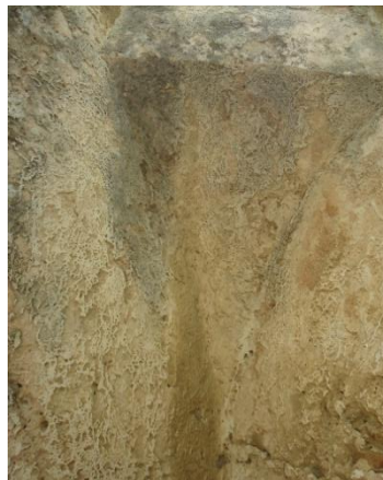
Figure 4.138. South East pendentive plaster of Cleaning Cell
