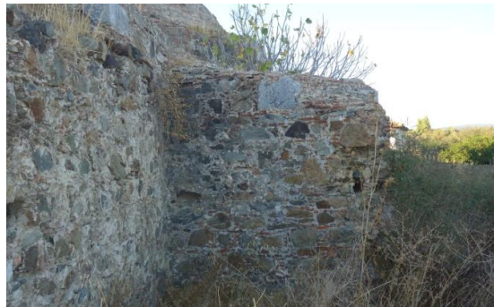
Figure 4.12. South wall - 2 of Düzce Bath
