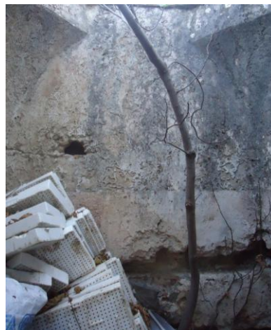
Figure 4.135. South wall plaster of Cleaning Cell
