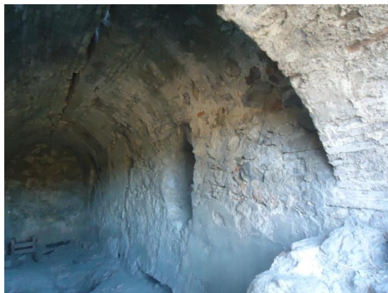
Figure 4.180. North wall of the water reservoir
