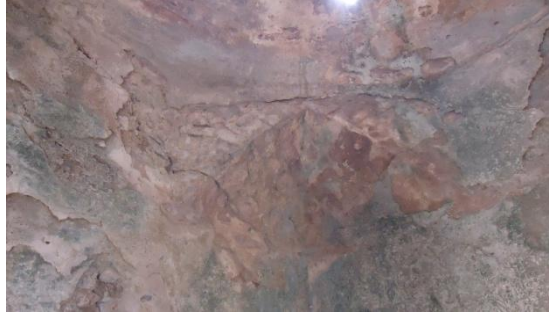
Figure 4.158. South East plane triangles plaster of the South East Halvet
