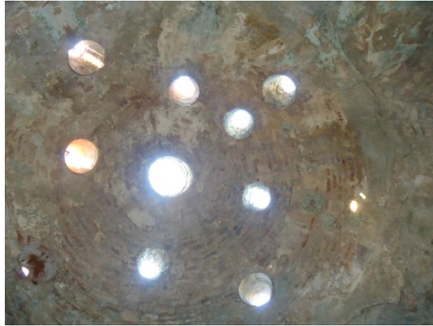
Figure 4.160. Dome plaster of the South East Halvet
