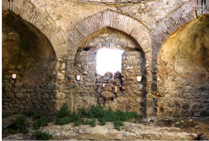
Figure 4.63. North Wall Plaster of Soyunmalik
