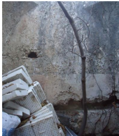
Figure 4.125. South wall of Cleaning Cell
