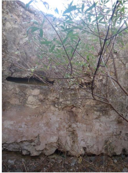
Figure 4.161. West wall of the South West Halvet
