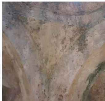
Figure 4.114. North East Pendentive plaster of Sıcaklık
