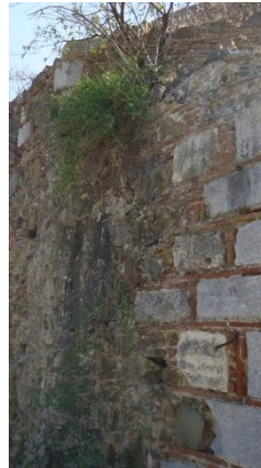
Figure 4.9. Plants on East wall - 1
