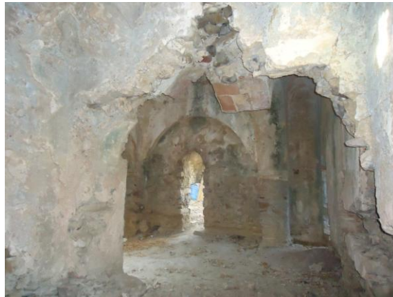
Figure 4.153. North wall plaster of the South East Halvet
