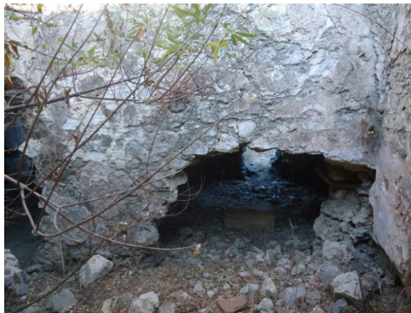
Figure 4.172. East wall plaster of the South West Halvet
