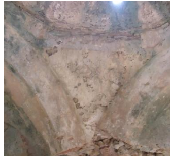
Figure 4.115. South East Pendentive of Sıcaklık
