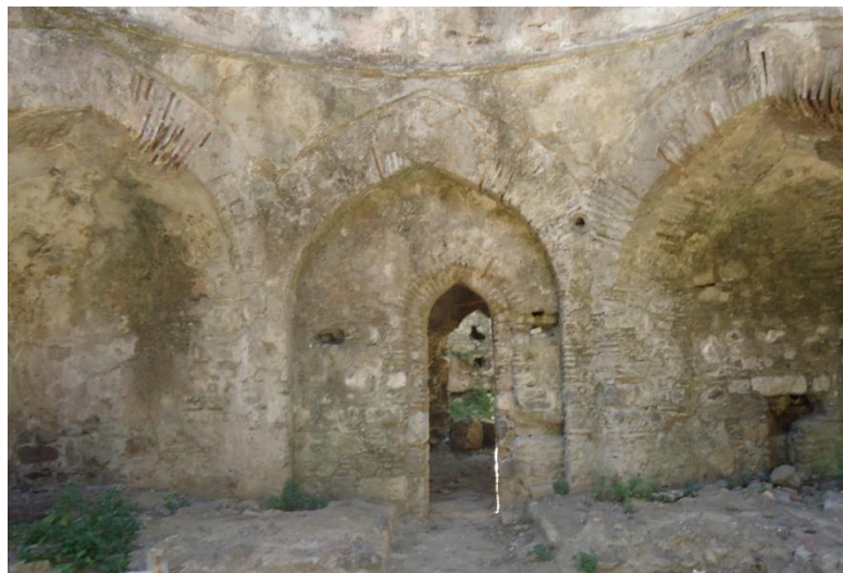
Figure 4.33. South wall of Soyunmalik
