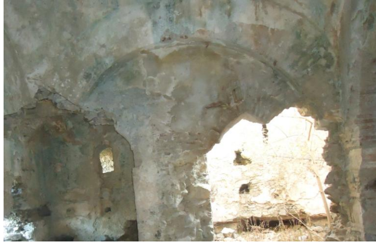
Figure 4.95. South Arch of Sicaklık
