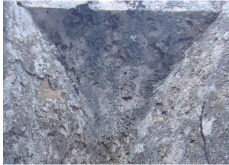
Figure 4.137. North East pendentive plaster of Cleaning Cell
