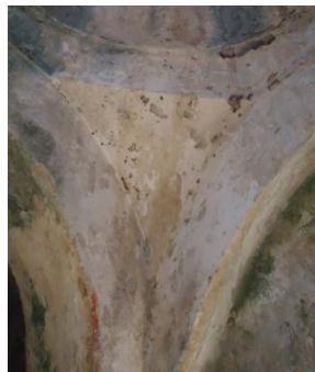
Figure 4.96. North West Pendentive of Sicaklık
