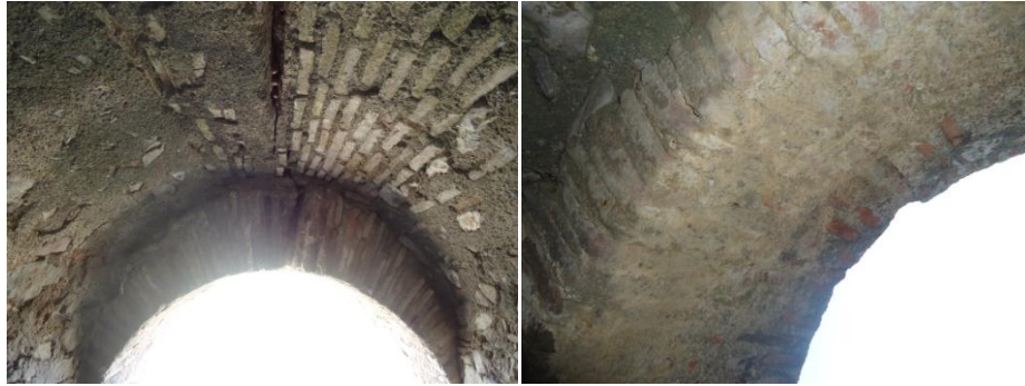
Figure 4.182. East arch of water reservoir
