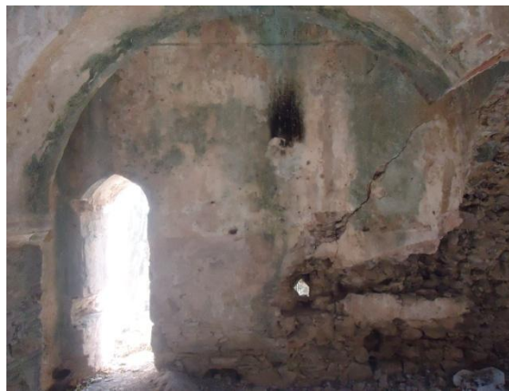
Figure 4.107. East Wall plaster of Sicaklık
