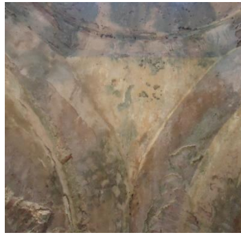
Figure 4.99. South West Pendentive of Sıcaklık
