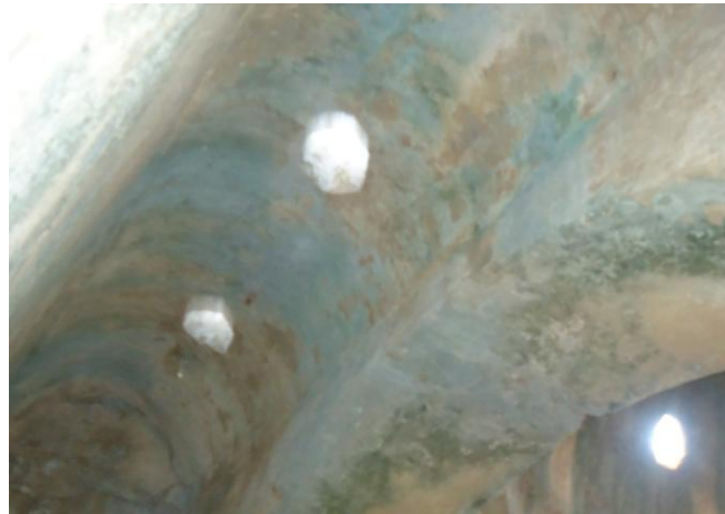
Figure 4.121. East Barrel Vault plaster of Sıcaklık
