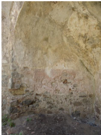
Figure 4.32. Right part of the East wall
