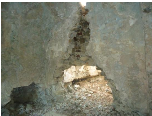
Figure 4.142. West wall of the South East Halvet
