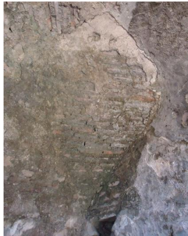
Figure 4.51. South West squinch of Soyunmalık
