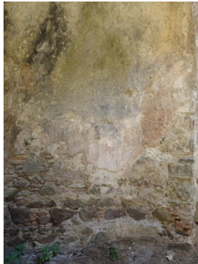
Figure 4.30. Left part of the East wall
