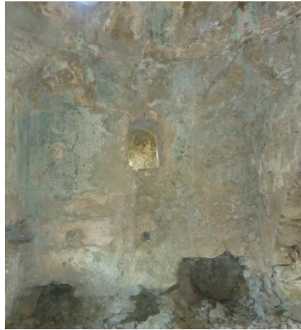
Figure 4.146. South wall of the South East Halvet
