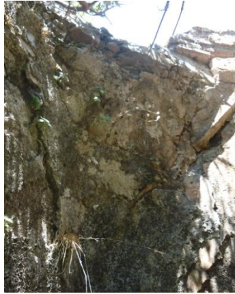
Figure 4.174. North West pendentive plaster of the South West Halvet
