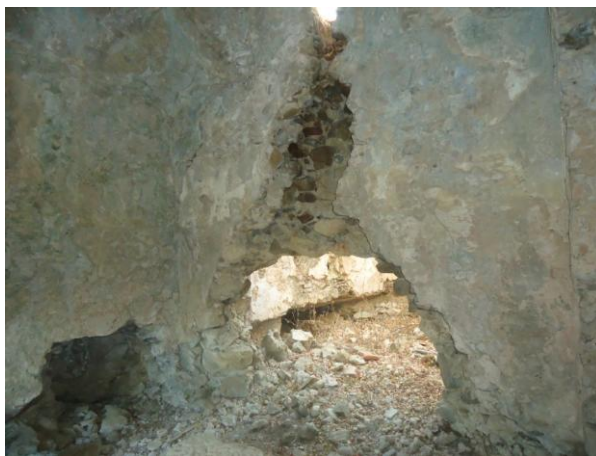
Figure 4.152. West wall plaster of the South East Halvet
