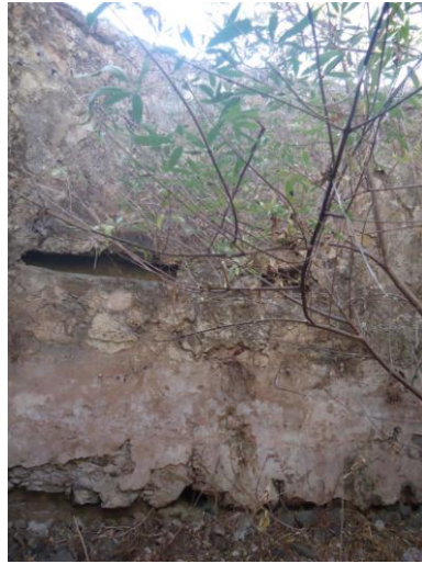
Figure 4.170. West wall plaster of the South West Halvet
