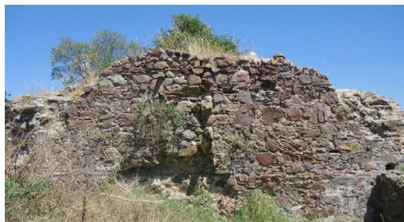
Figure 4.11. South wall - 1 of Düzce Bath
