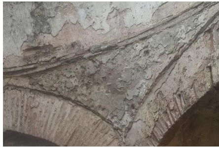
Figure 4.80. North East plane triangle - 1 plaster of Soyunmalık
