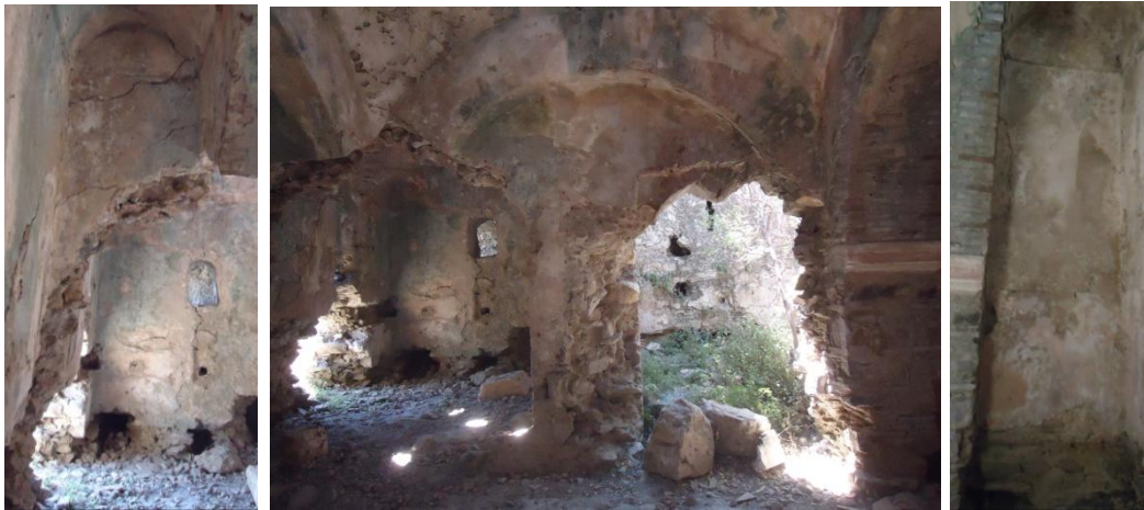
Figure 4.91. South Wall of Sıcaklık
