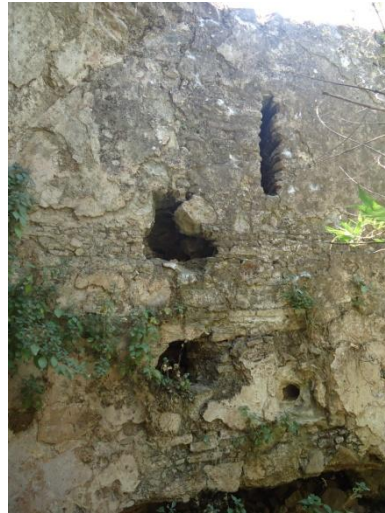
Figure 4.173. South wall plaster of the South West Halvet
