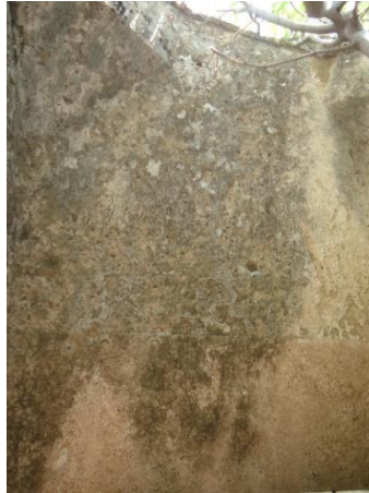
Figure 4.134. East wall plaster of Cleaning Cell
