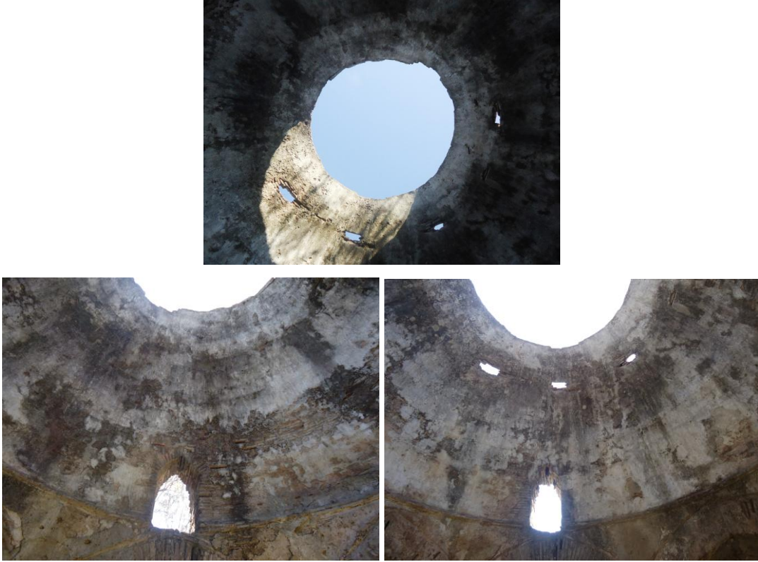
Figure 4.86. Dome plaster of Soyunmalik
