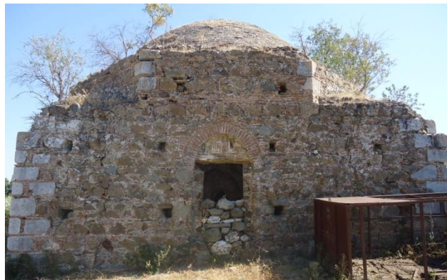
Figure 4.6. North wall - 1 of Düzce Bath
