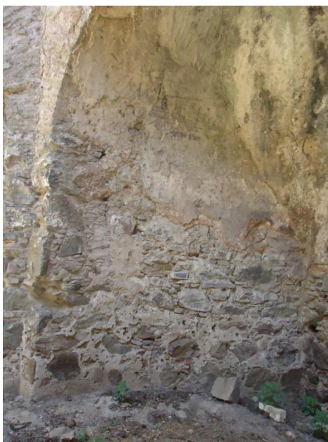
Figure 4.28. Right part of the North wall
