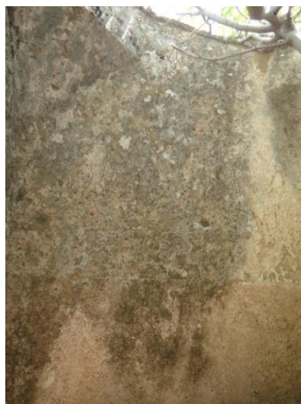
Figure 4.124. East wall of Cleaning Cell
