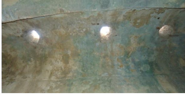
Figure 4.120. West Barrel Vault plaster of Sıcaklık
