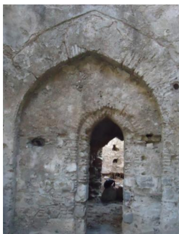
Figure 4.72. South arch plaster of Soyunmalik
