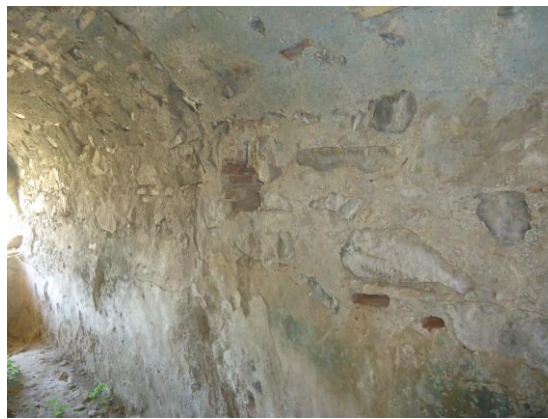
Figure 4.181. South wall of water reservoir
