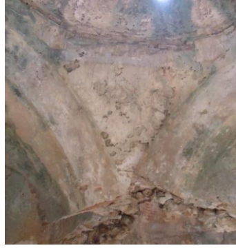
Figure 4.98. South East Pendentive of Sıcaklık
