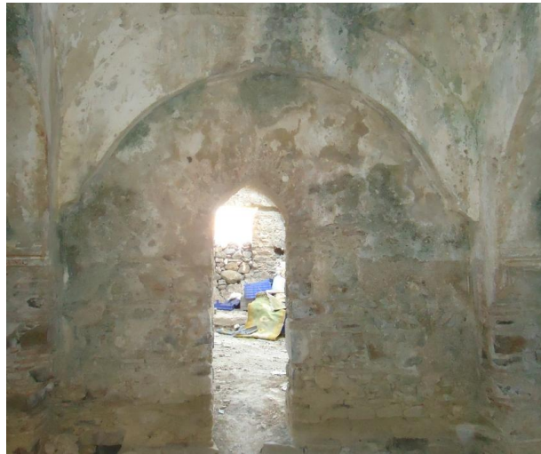
Figure 4.110. North Arch plaster of Sıcaklık
