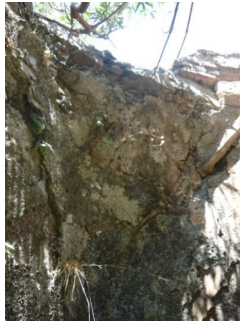
Figure 4.165. North West pendentive of the South West Halvet
