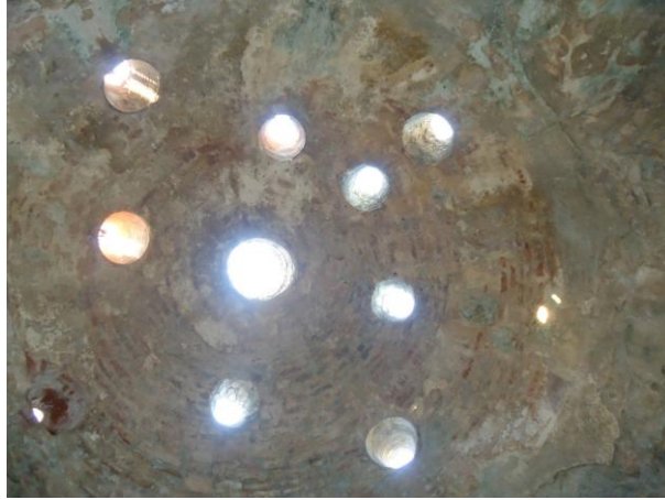
Figure 4.151. Dome of South East Halvet
