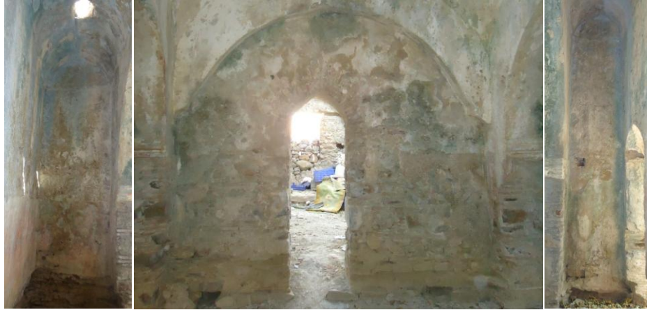
Figure 4.89. North Wall of Sicaklık
