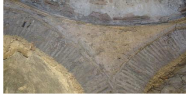
Figure 4.79. North West plane triangle plaster- 2 of Soyunmalık
