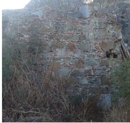
Figure 4.10. East wall - 2 of Düzce Bath
