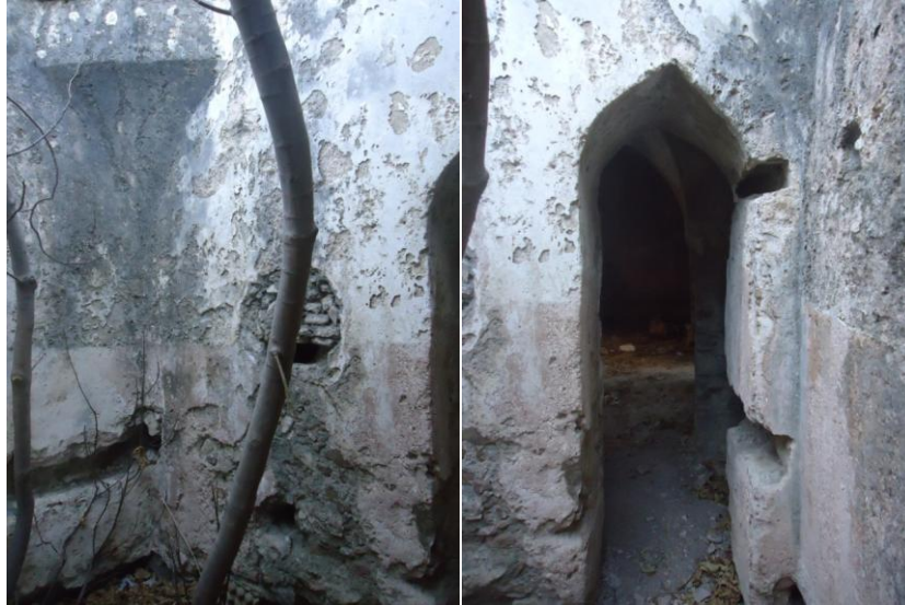
Figure 4.122. West wall of Cleaning Cell
