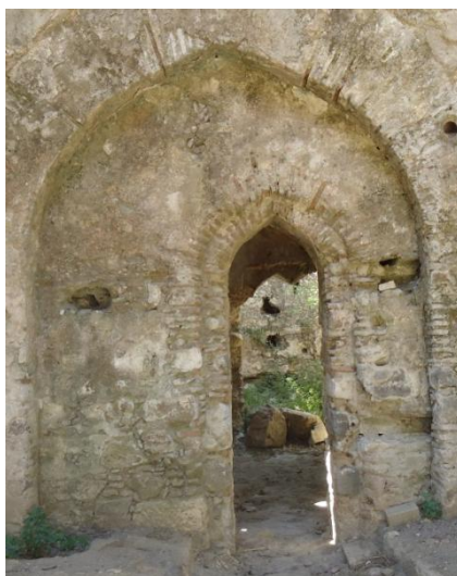
Figure 4.35. Middle part of the South wall
