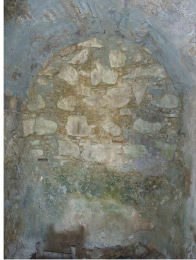
Figure 4.179. West wall of the water reservoir
