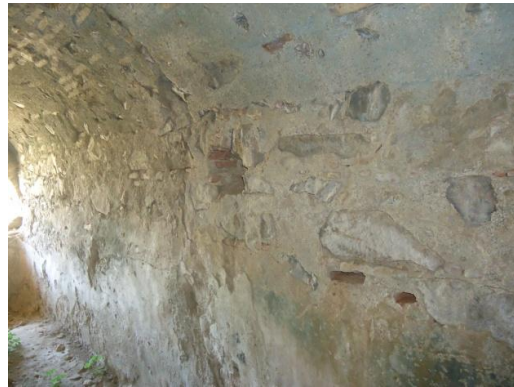
Figure 4.186. South wall plaster of the water reservoir
