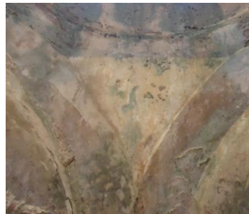
Figure 4.116. South West Pendentive plaster of Sıcaklık
