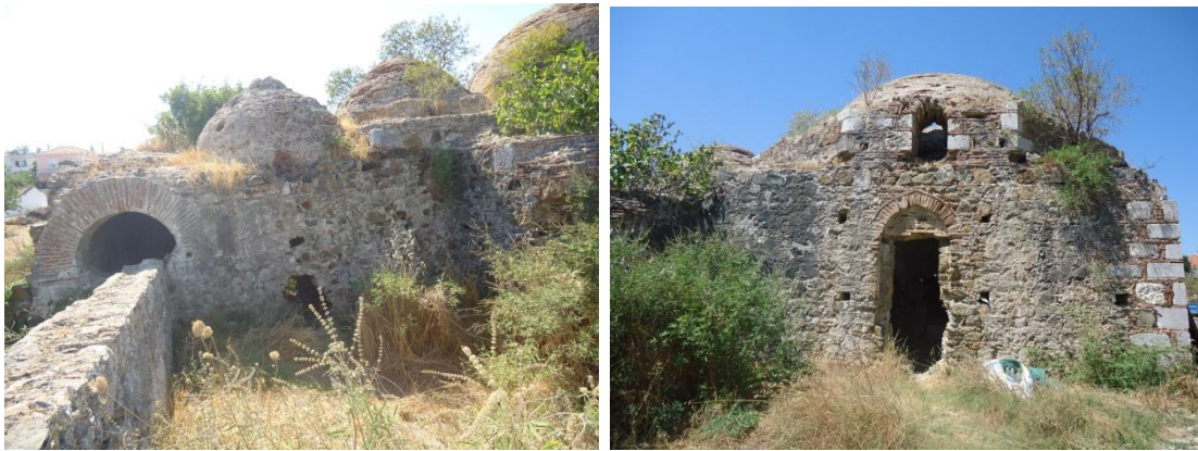
Figure 4.8. East wall - 1 of Düzce Bath
