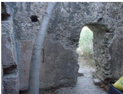
Figure 4.123. North wall of Cleaning Cell
