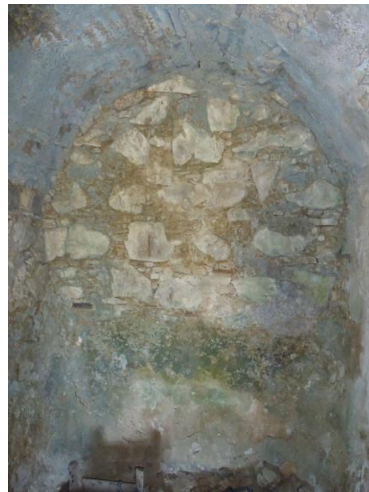
Figure 4.184. West wall plaster of the water reservoir
