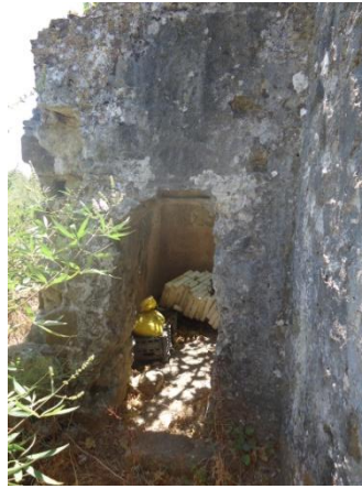
Figure 4.8. North wall - 2 of Düzce Bath
