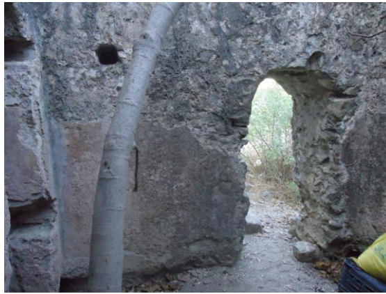
Figure 4.133. North wall plaster of Cleaning Cell
