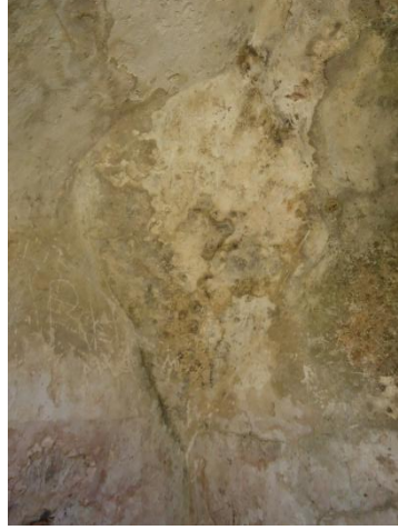
Figure 4.76. South East squinch plaster of Soyunmalik
