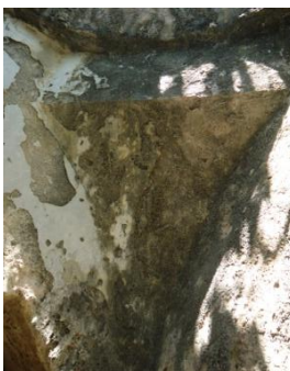
Figure 4.126. North West pendentive of Cleaning Cell
