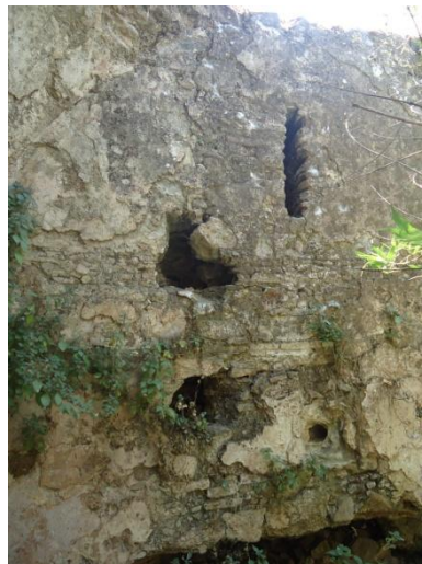
Figure 4.164. South wall of the South West Halvet
