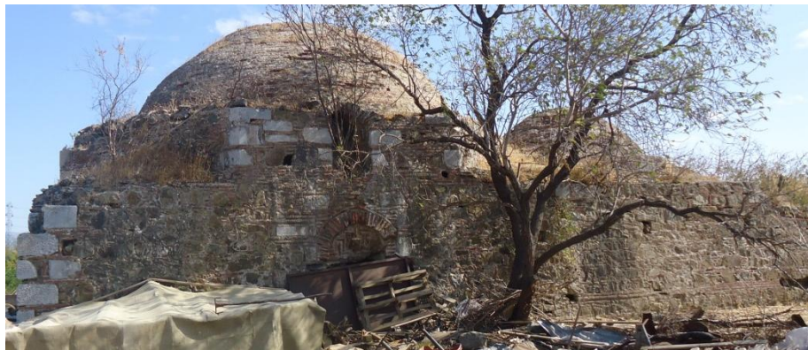
Figure 4.4. West wall of Düzce Bath
