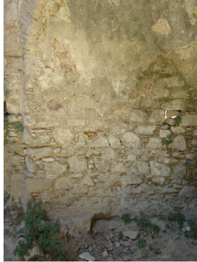
Figure 4.22. Right part of the West wall
