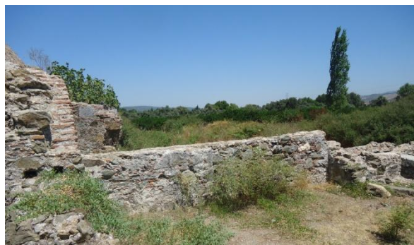
Figure 4.15. The wall (between cistern and water reservoir)
