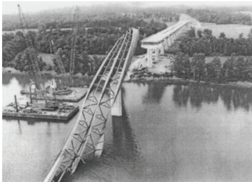
Figure 2.2. Tennessee River Bridge on the day of collapse. (Source: https://failures.wikispaces.com/Tennessee+River+Bridge+Collapse ).
