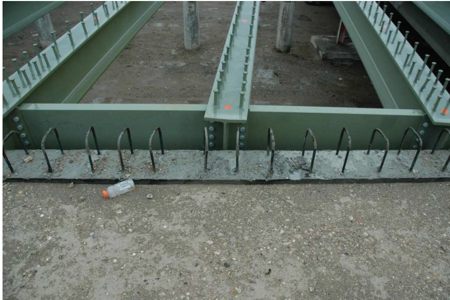
Figure 3. 10. Transverse diaphragm at the supports.
