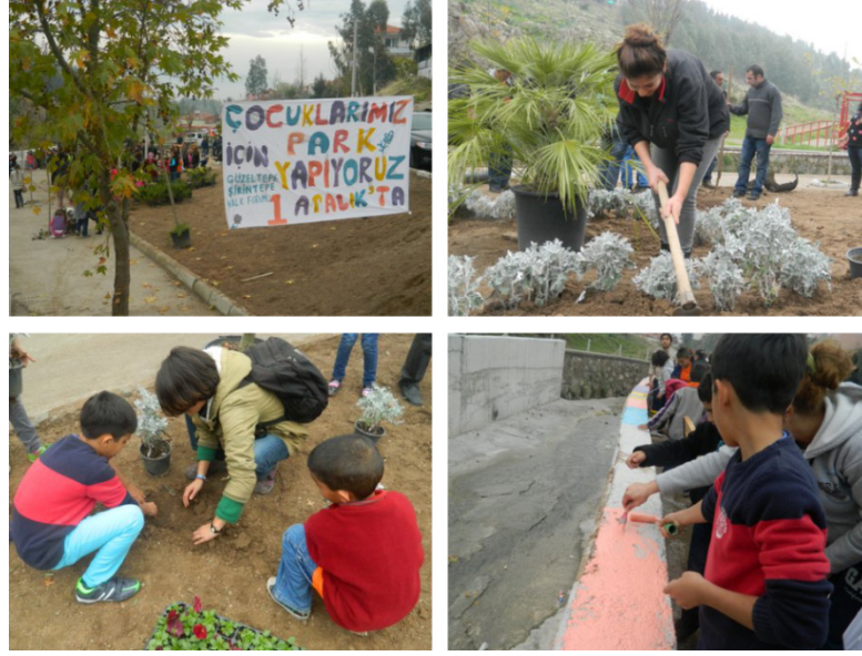
Figure 4.16. Views During Park Construction in Güzeltepe - Çiğli/İzmir (Source: Halkevleri, 2013c)
