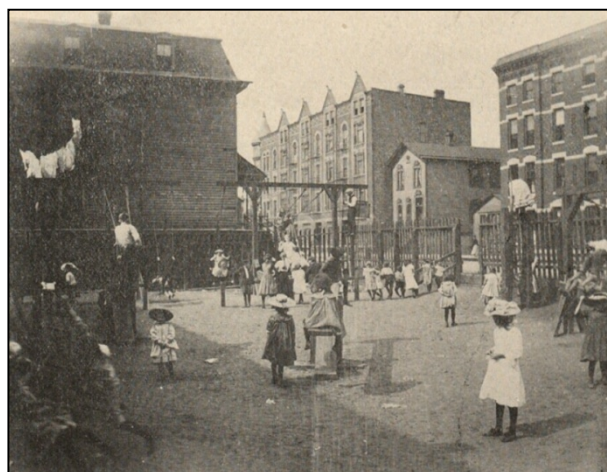
Figure 3.2. The Playground, an essential part of early twentieth-century social reform (Source: Talen, 2015)
