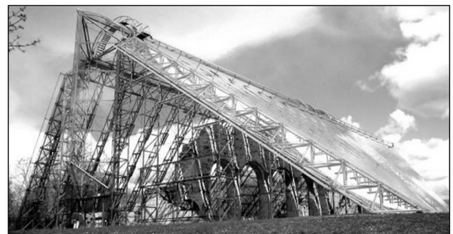
Fig. 5. Protective enclosure over the Hamar Cathedral, Norway [24].
