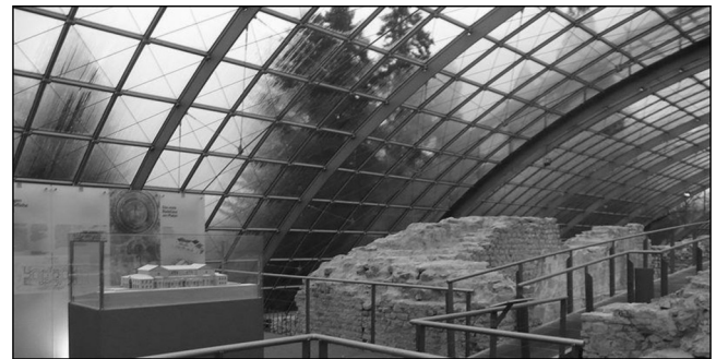
Fig. 4. Condensation on the glass, Badenweiler, Germany [23].
