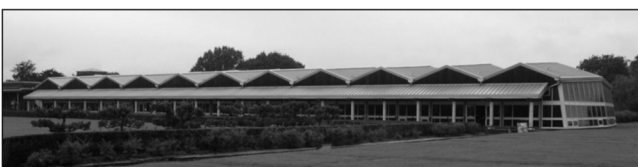
Fig. 2. Protective enclosure over the Roman Villa Fishbourne Roman Palace at West Sussex, England [22].
