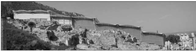
Fig. 6. Protective enclosure over the Terrace Houses 2 at Ephesus, Turkey.
