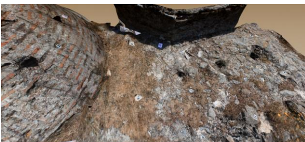
Figure 20. Detailed part of North West in superstructure
