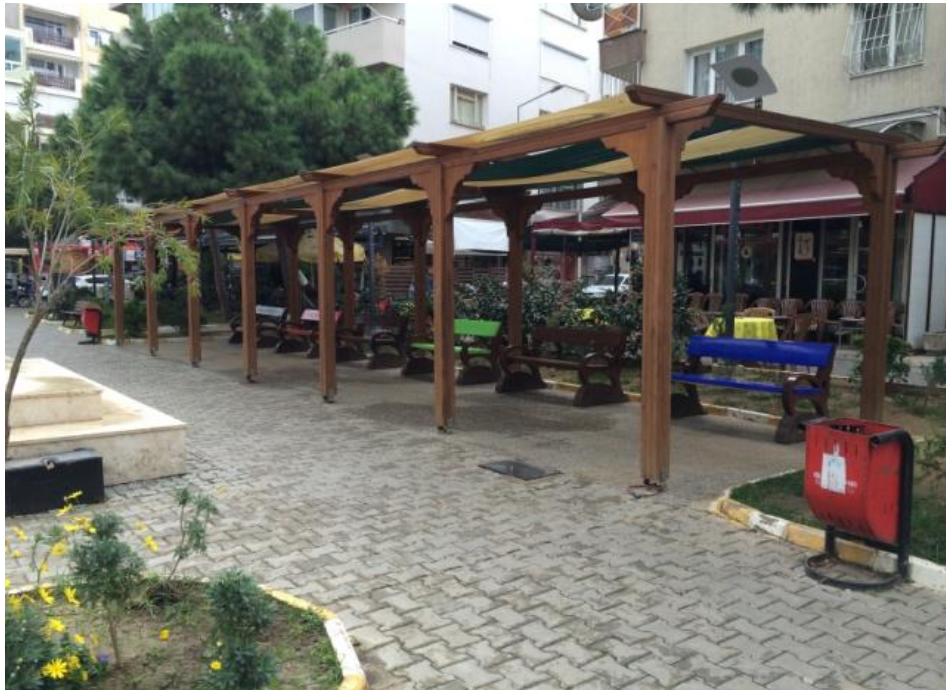
Figure 62. Duru Park shading element with inappropriate material
