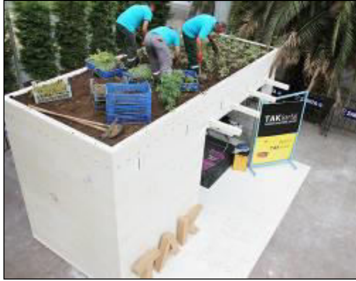
Figure 3.22. TAK Kondu in Kartal Square, Istanbul (Source: TAK, 06.09.2015)
