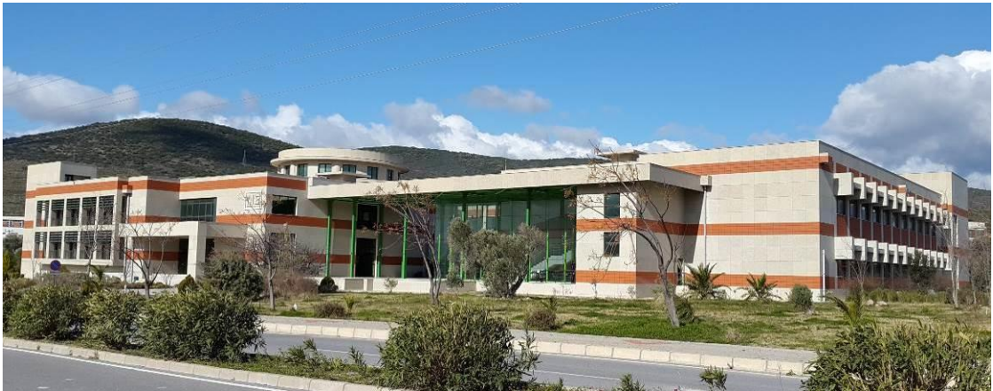
Figure 3.2 View from main entrance (Southeast façade) of the building
