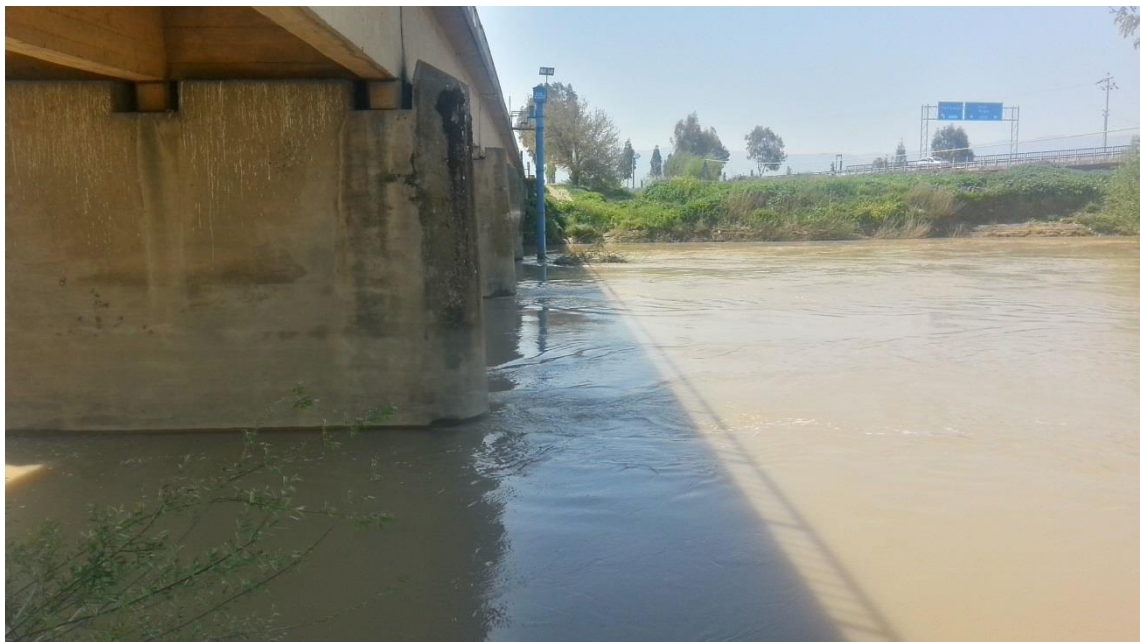
Figure 5.35. A view of turbulence effect of piers on B. Menderes River
