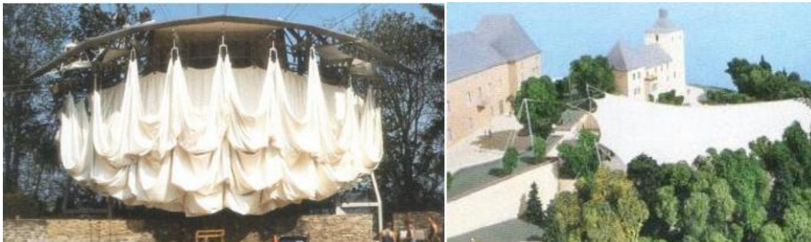
Figure 3.31. Cable membrane roof for the open-air theatre in Wiltz, Luxemburg (Source: Otto & Rasch, 1995).
