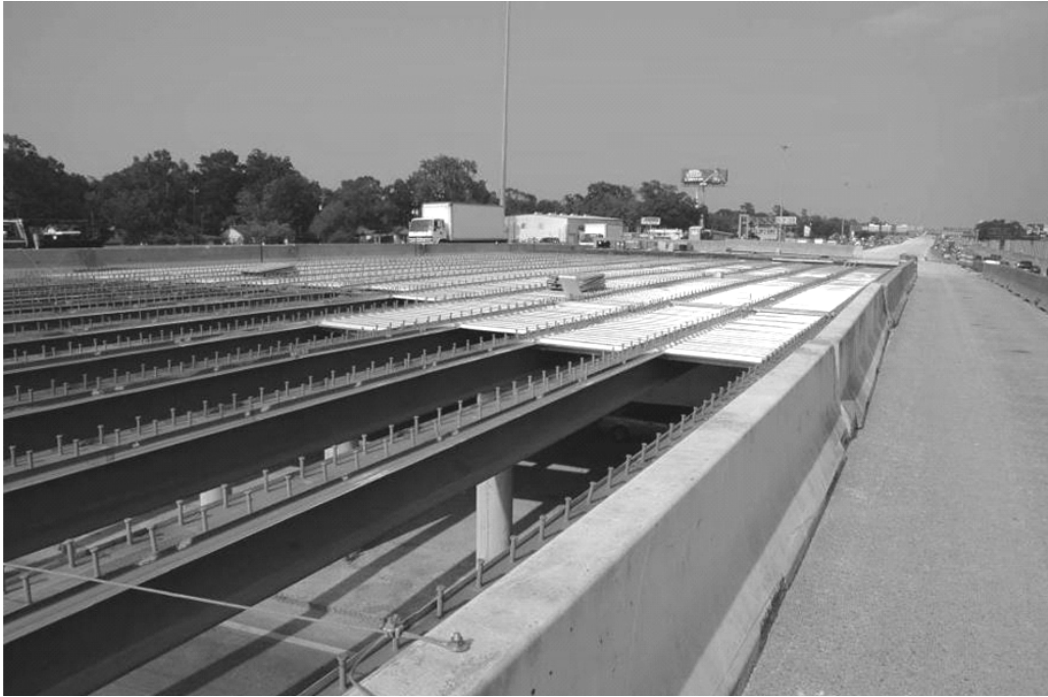
Figure 1.3. Diaphragm bracing implementation from Houston, TX, USA
