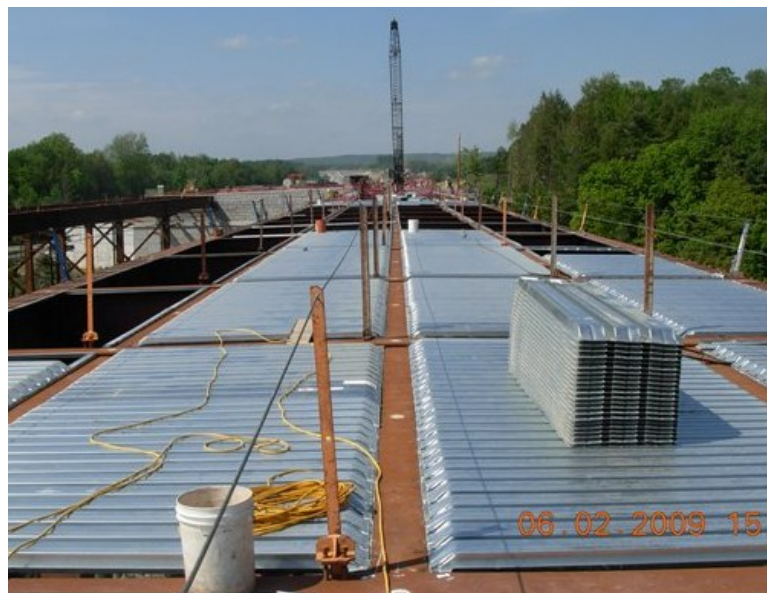
Figure 1.5. PMDF in bridge industry (Source: New York State Department of Transportation [NYSDOT], 2009)
