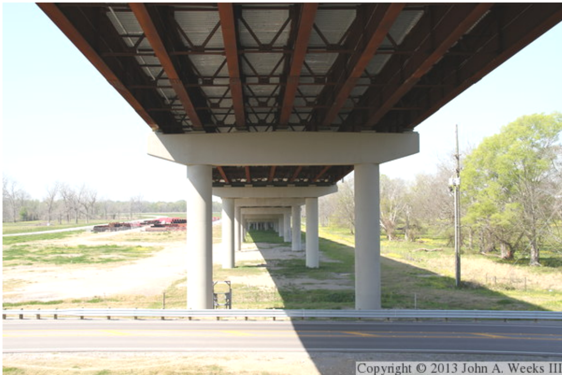
Figure 1.2. Intermediate discrete braces with metal deck forms (Source: Weeks, 2013)
