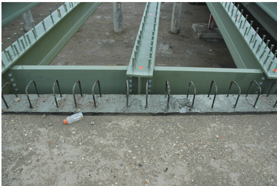
Figure 3.6 Transverse diaphragm between the girders
