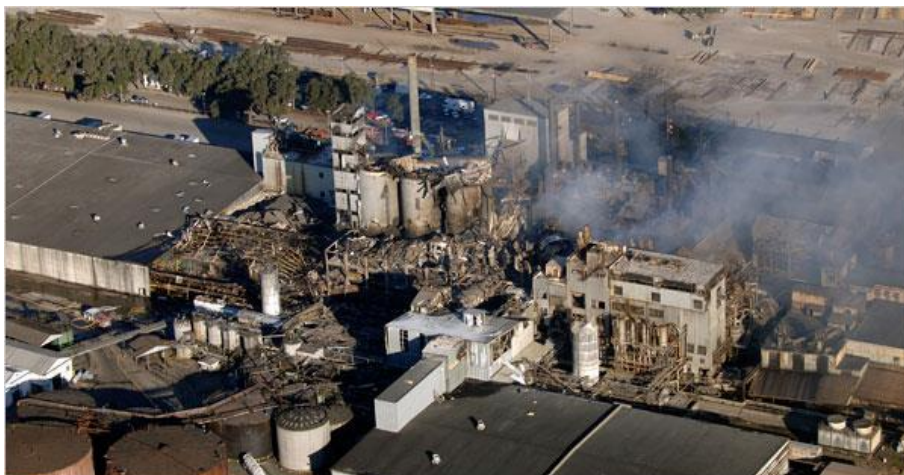
Figure 2.4. An explosion at a sugar refinery due to ESD in Georgia (US) (Source: Explosion due to ESD 2011)
