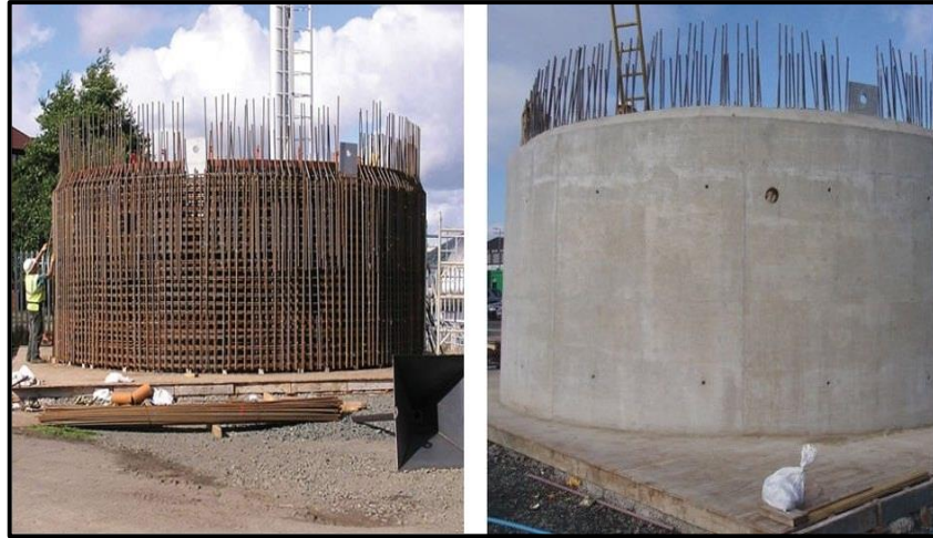
Figure 2.4. Dense steel reinforcement building [5]
