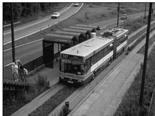
Figure 2.23 Bus Stop Reached from Roads
