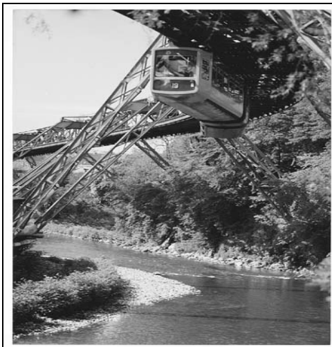
Figure 2.3 Wuppertal Monorail System
