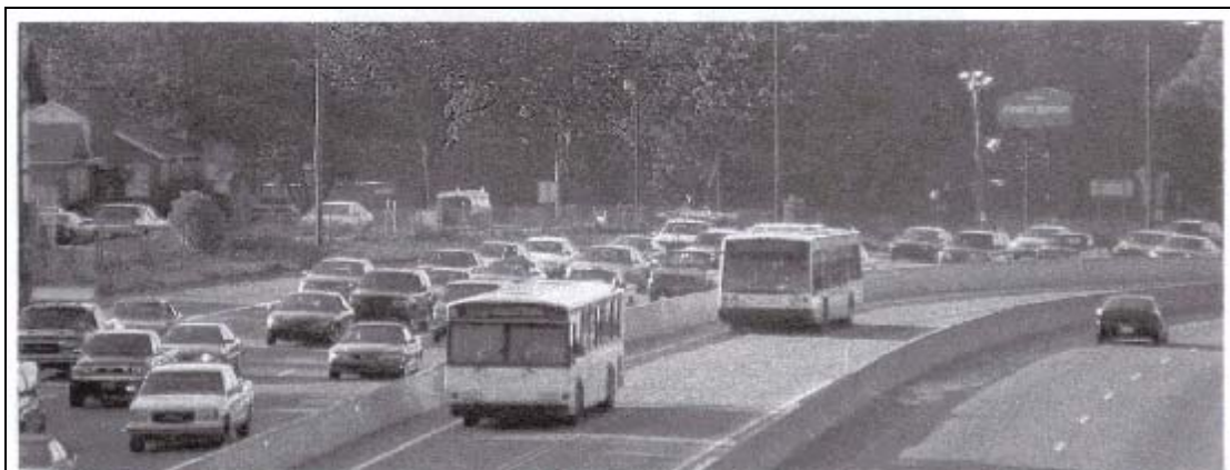
Figure 4.4 Busway in Charlotte, NC
