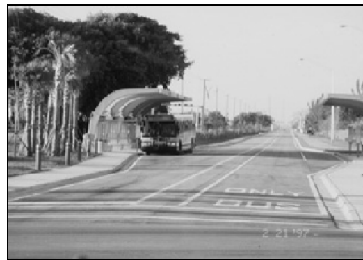
Figure 4.18 Side-Aligned At-Grade Busway Miami, FL
