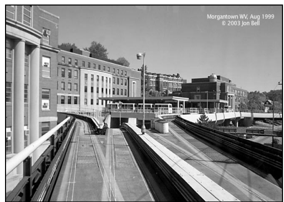
Figure 2.8 The Elevated Concrete Guideway
