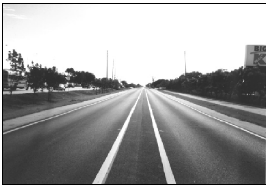
Figure 4.17 Side-Aligned At-Grade Busway Miami, FL
