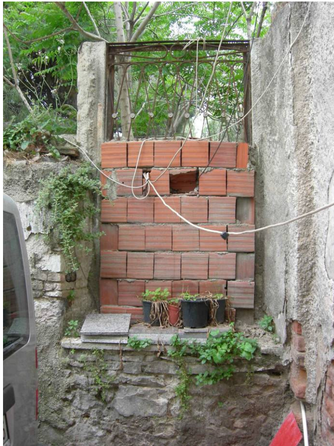
Figure 4.2. The original wall piece at the south of the annex.
