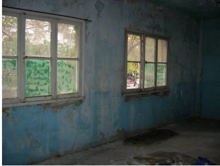
Figure 2.112. The additional rooms of the annex at the mezzanine floor.
