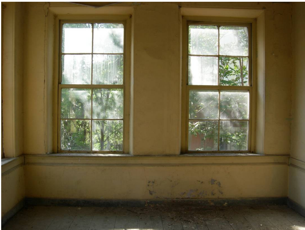
Figure 2.65. The timber sash windows of room 4 at the first floor.
