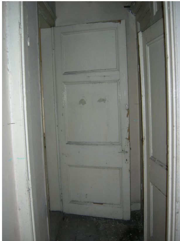
Figure 2.71. The door between the stair hall and the connection space.
