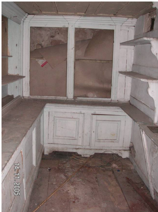
Figure 2.101. The east wall of the kitchenette.
