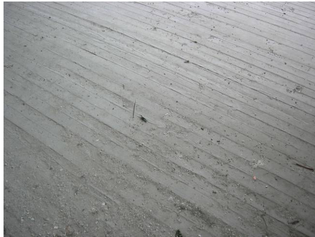
Figure 2.77. The floor covering of room 6 at the first floor.
