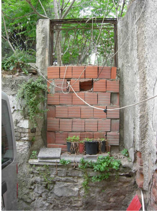
Figure 2.106. The wall piece at the south of the annex.
