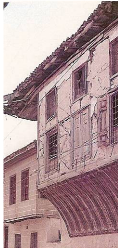
Figure 3.79. Timber skeleton with adobe infill. (Source: Bektaş 1996)
