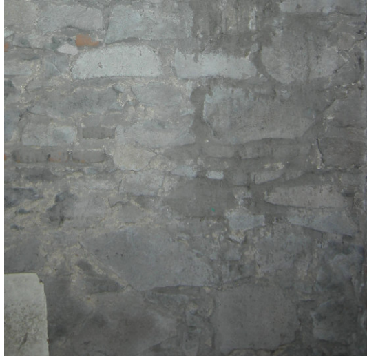
Figure 2.14. Exposed stone walls of Space 2 at the basement.
