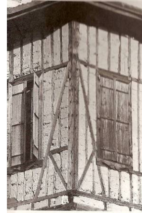
Figure 3.78. Timber skeleton with brick infill. (Source: Bektaş 1996).
