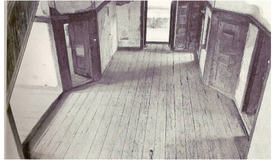
Figure 3.40. A central hall with chamfered corners. (Source: Kuban 1995)
