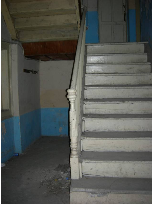
Figure 2.39. The halfpace timber stair.
