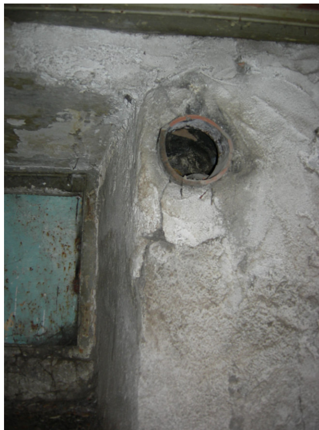
Figure 2.18. The ceramic pipe on the northern wall of wet space 2.
