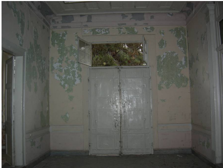
Figure 2.28. The northern wall of the inner hall at the ground floor.
