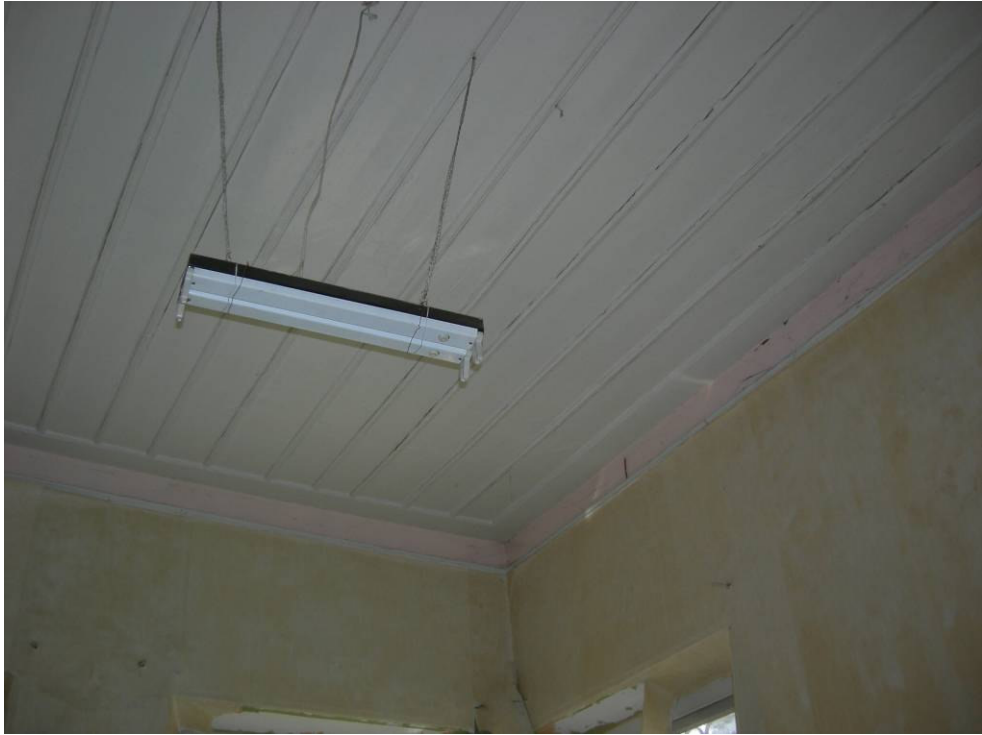
Figure 2.35. The ceiling of room 2.
