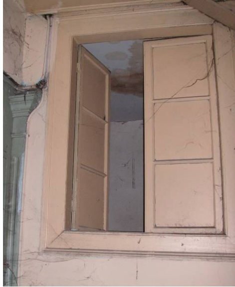
Figure 2.56. The interior window of the storage room at the mezzanine floor.
