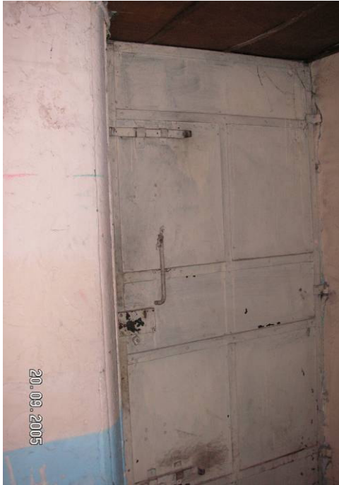
Figure 2.41. The iron door between the annex and the stairwell.
