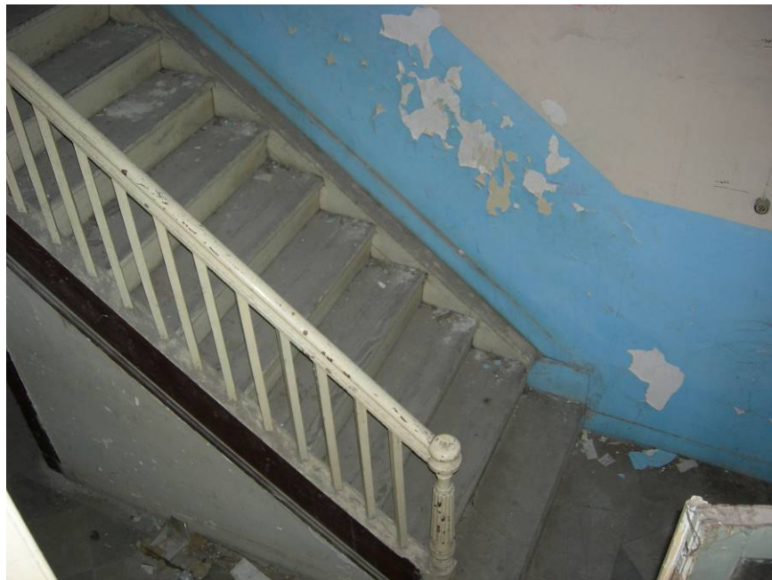
Figure 2.103. The half pace timber stair and its timber balustrade.
