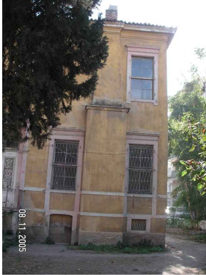
Figure 2.86. The projecting fireplace and the chimney at the northern facade.
