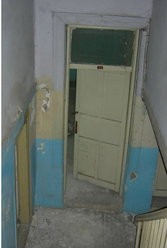
Figure 2.58. The door of the room 2 of the annex at the mezzanine level.
