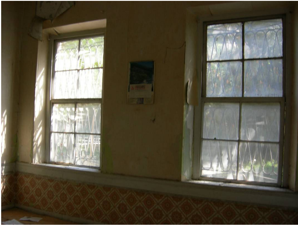
Figure 2.33. The windows on the southern wall of room 1.
