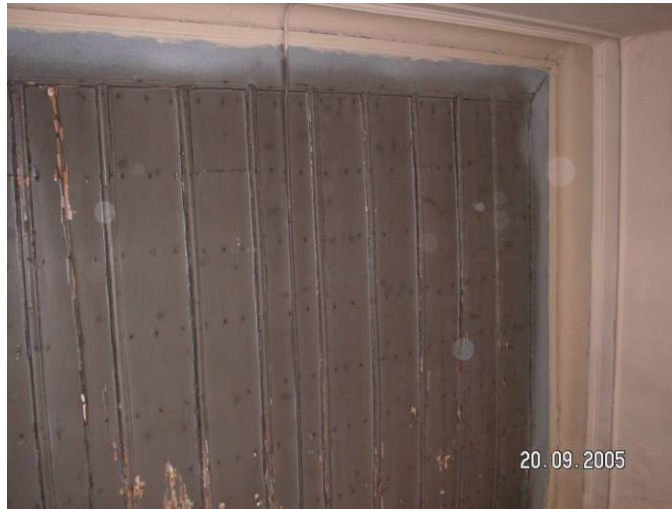
Figure 2.68. The ceiling covering of room 5 at the first floor.
