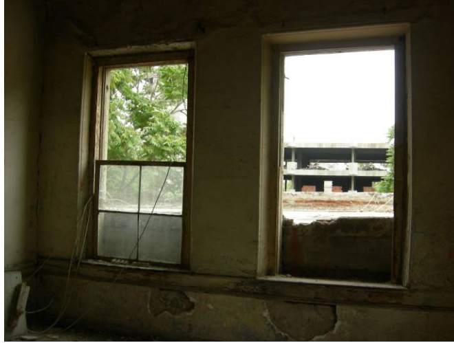
Figure 2.76. The eastern wall of room 6 at the first floor.
