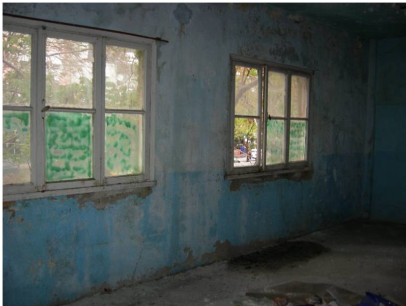
Figure 2.59. Room 2 of the annex at the mezzanine level.
