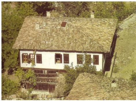
Figure 3.82. Hipped roof. (Source: Kuban 1995)
