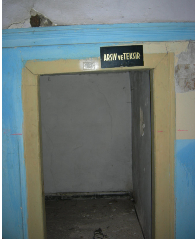
Figure 2.54. The entrance to the storage room at the mezzanine floor.
