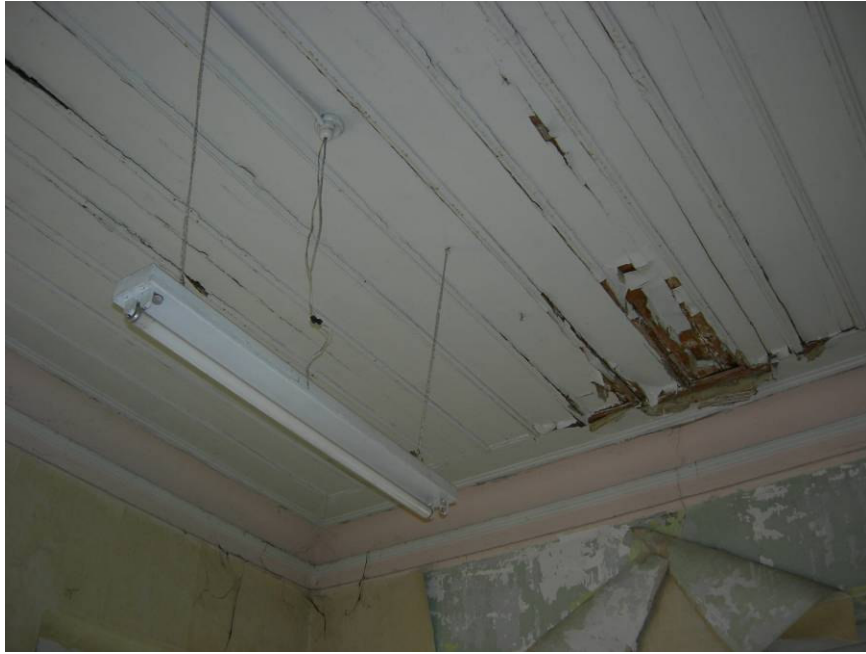
Figure 4.7. The ceiling of room1.
