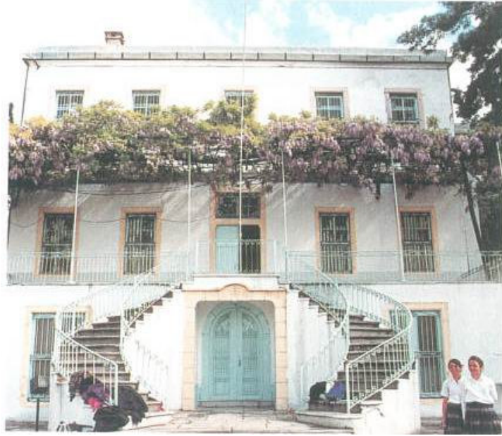
Figure 3.102. Latife Hanım House in Köprü. ( Source: Kabaoğlu et al. 1999)
