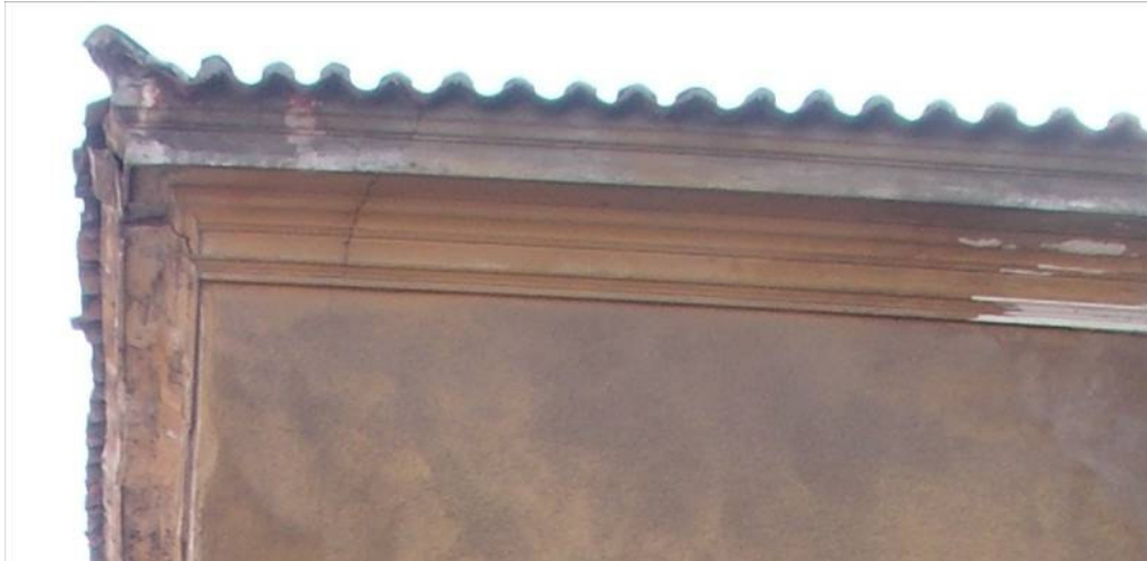
Figure 2.104. The roof cornice of the house.
