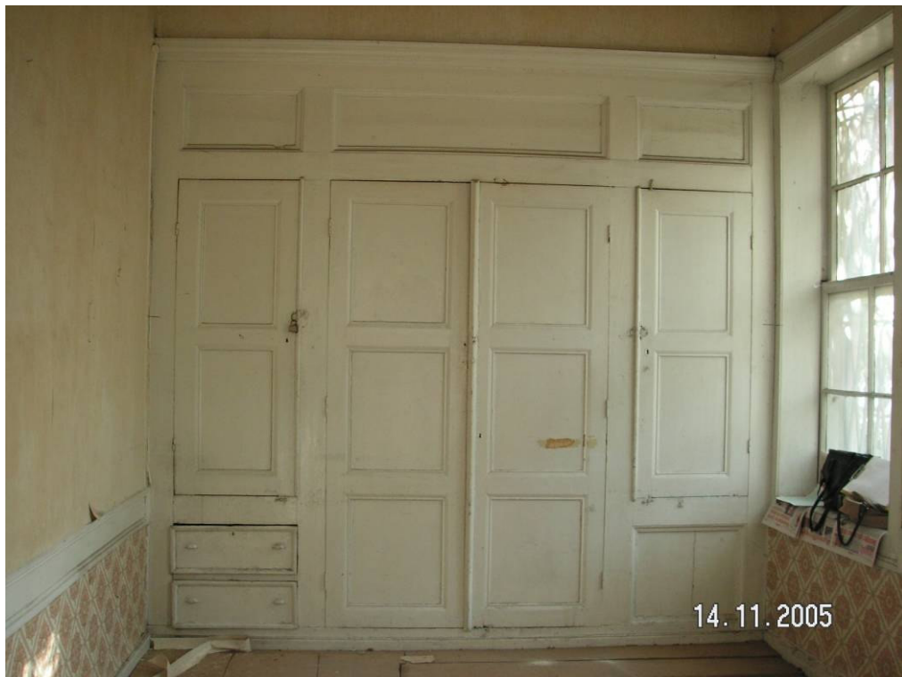
Figure 2.47. The cupboard in room 3.
