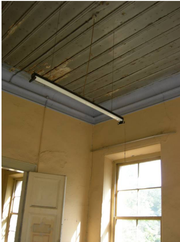
Figure 2.64. The ceiling and the moldings in room 4 at the first floor.
