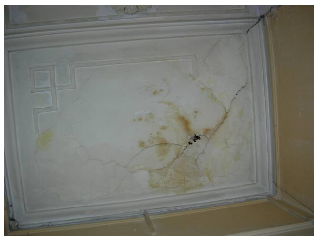
Figure 2.70. The ceiling of the stair hall at the first floor.
