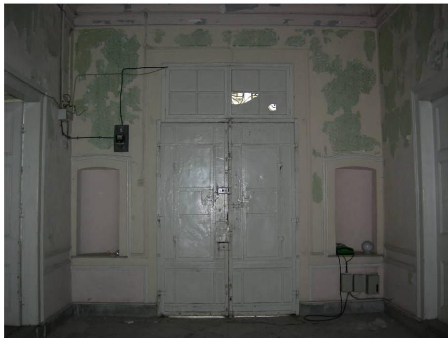
Figure 2.26. The southern wall of the hall and its elements.
