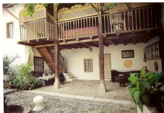
Figure 3.22. The hall at the ground floor. (Source: Günay 1997)
