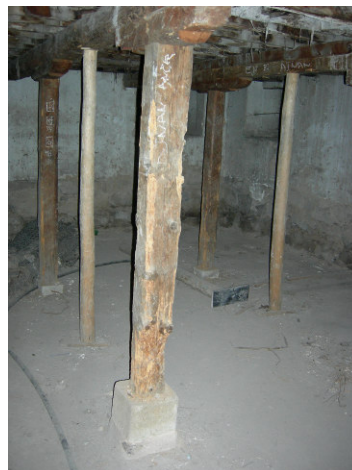
Figure 2.11. The supporting studs in the western part of the basement.
