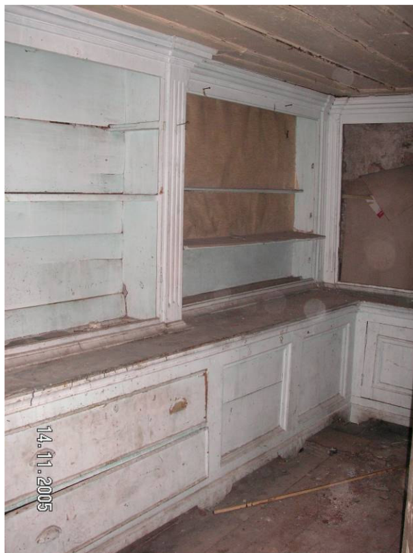
Figure 2.45. Cupboards of the kitchenette.
