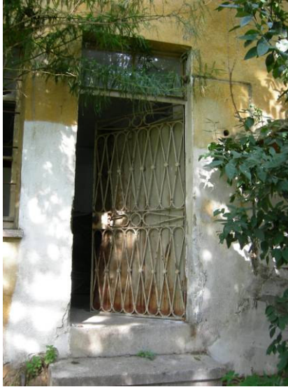
Figure 2.51. The door of the annex.
