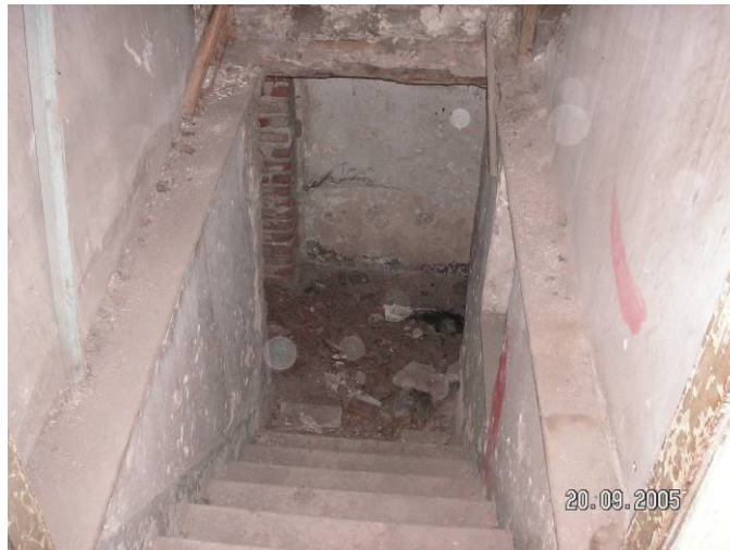
Figure 2.10. The stairs leading to the eastern part of basement.
