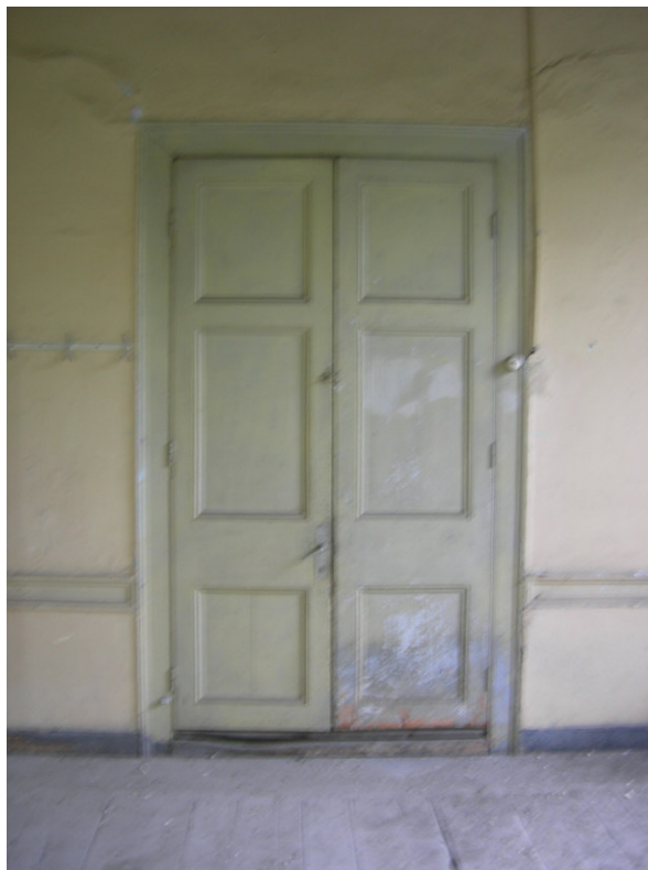
Figure 2.67. The door providing entrance to room 5 at the first floor.
