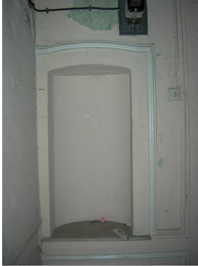
Figure 2.102. The semi circular niche on the south wall of the hall at the ground floor.
