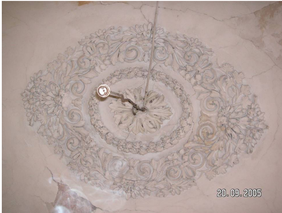
Figure 2.60. The stucco work in the center of the ceiling of the hall at the first floor.
