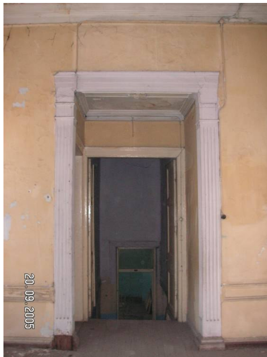
Figure 2.63. The pilasters at the first floor.
