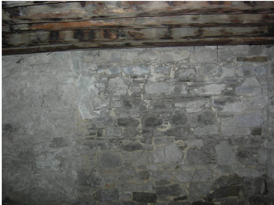
Figure 2.107. The masonry walls of the house at the basement.
