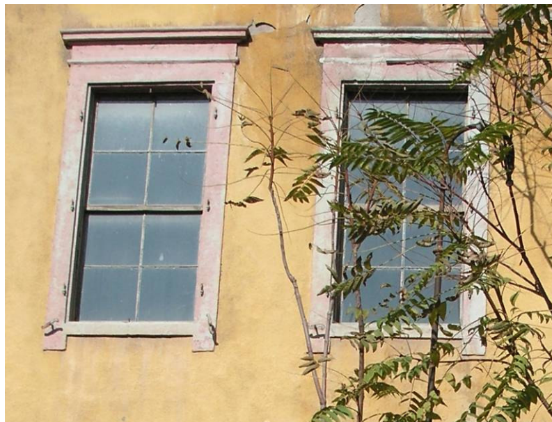
Figure 2.82. Timber sash windows with stone casings at the first floor level.
