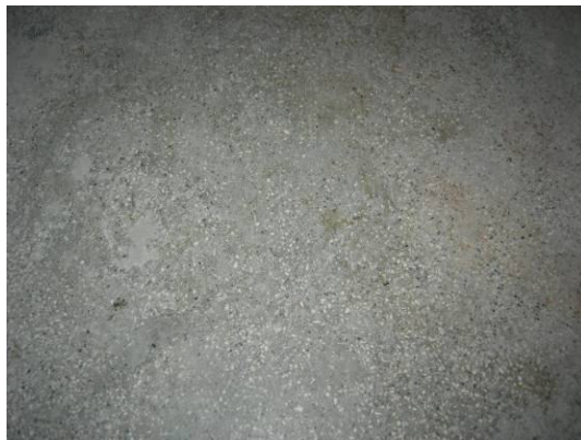
Figure 2.53. The floor covering of the annex.
