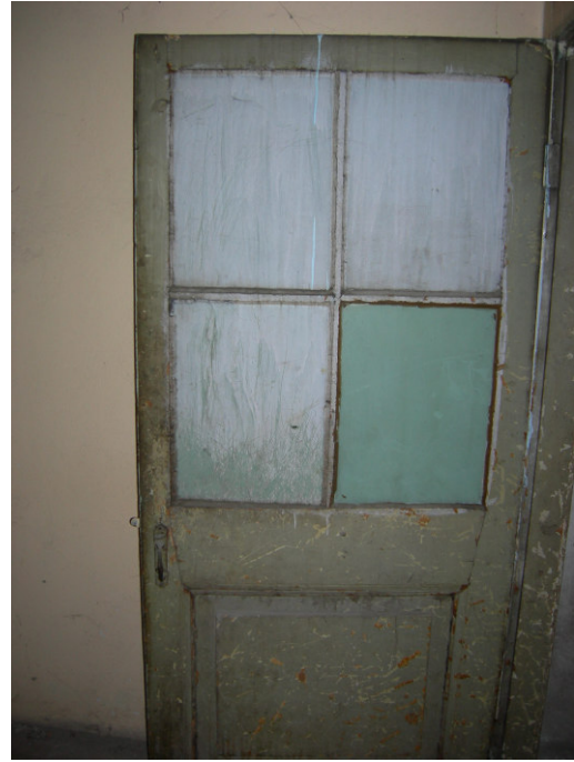
Figure 2.42. The door providing entrance to the stairs leading to the basement.
