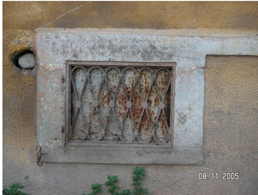
Figure 4.5. Shutter backstops of the windows of wet space 1 and 2 at the basement.
