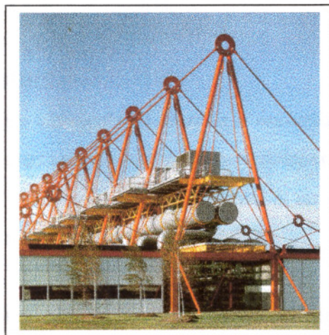
Figure 4. 39. The Laboratories and Corporate Facility for PA Technology building (source: Davies, 1991)
