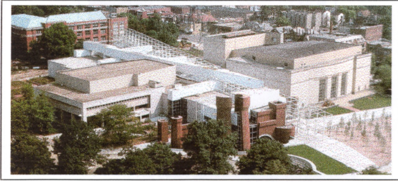
Figure 4. 46. Wexner Centre for the Visual Arts (source: Steele, 1997)
