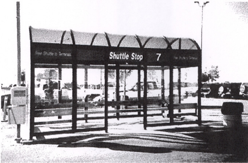
Figure 4.21. Acrylic is Used for Roof on Shelters ( http://www.sieger-design.de )
