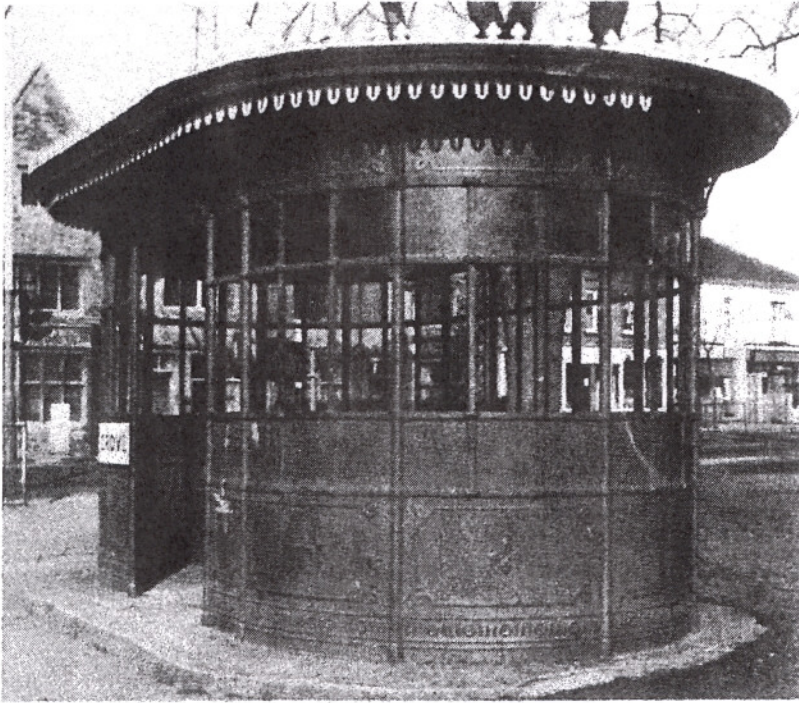
Figure 2.8. Iron Passenger Shelter in Northampton (Aaron, 1991, p.30)
