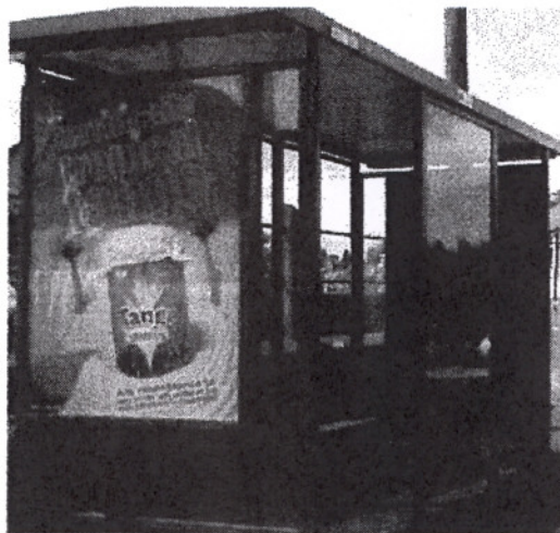
Figure 4.7. Shelter in Northern Climate with Two Openings for Entering and Exiting (Texas Transportation Institute, 1996, p. Appendix E-20)
