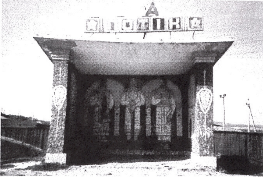
Figure 4.18. Concrete Bus Stop ( http://www.brama.com/travel/pics/bstop5.jpg )
