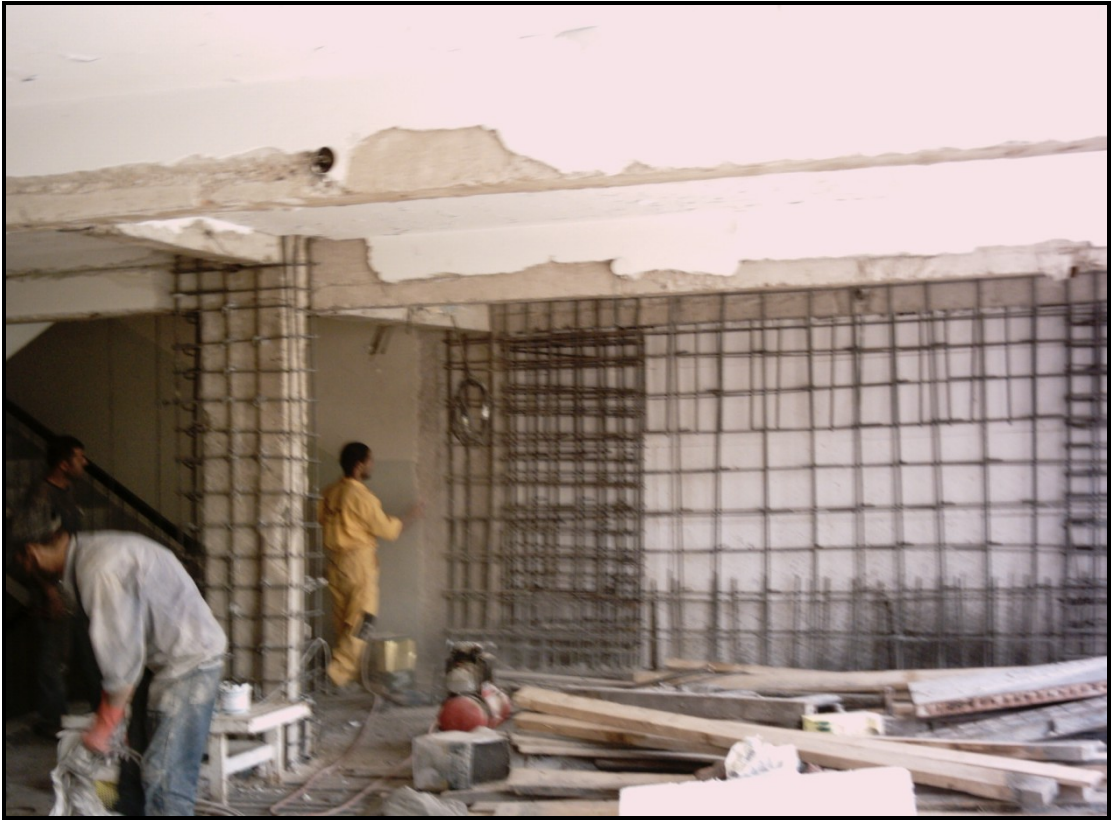
Figure 6.5. A New Shear Wall
