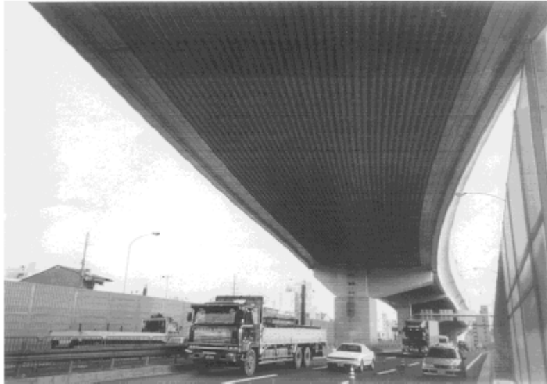
Figure 2.15. Foam layer used under an elevated viaduct as a noise insulator (Source: Miyoshi, et al. 2000)
