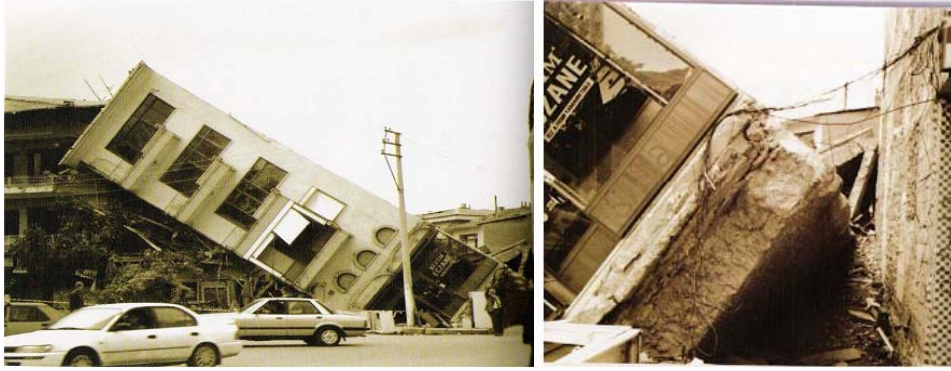
Figure 3.32. Pounding from Marmara earthquake due to the liquefaction (Source: Çiftçi, 1999)
