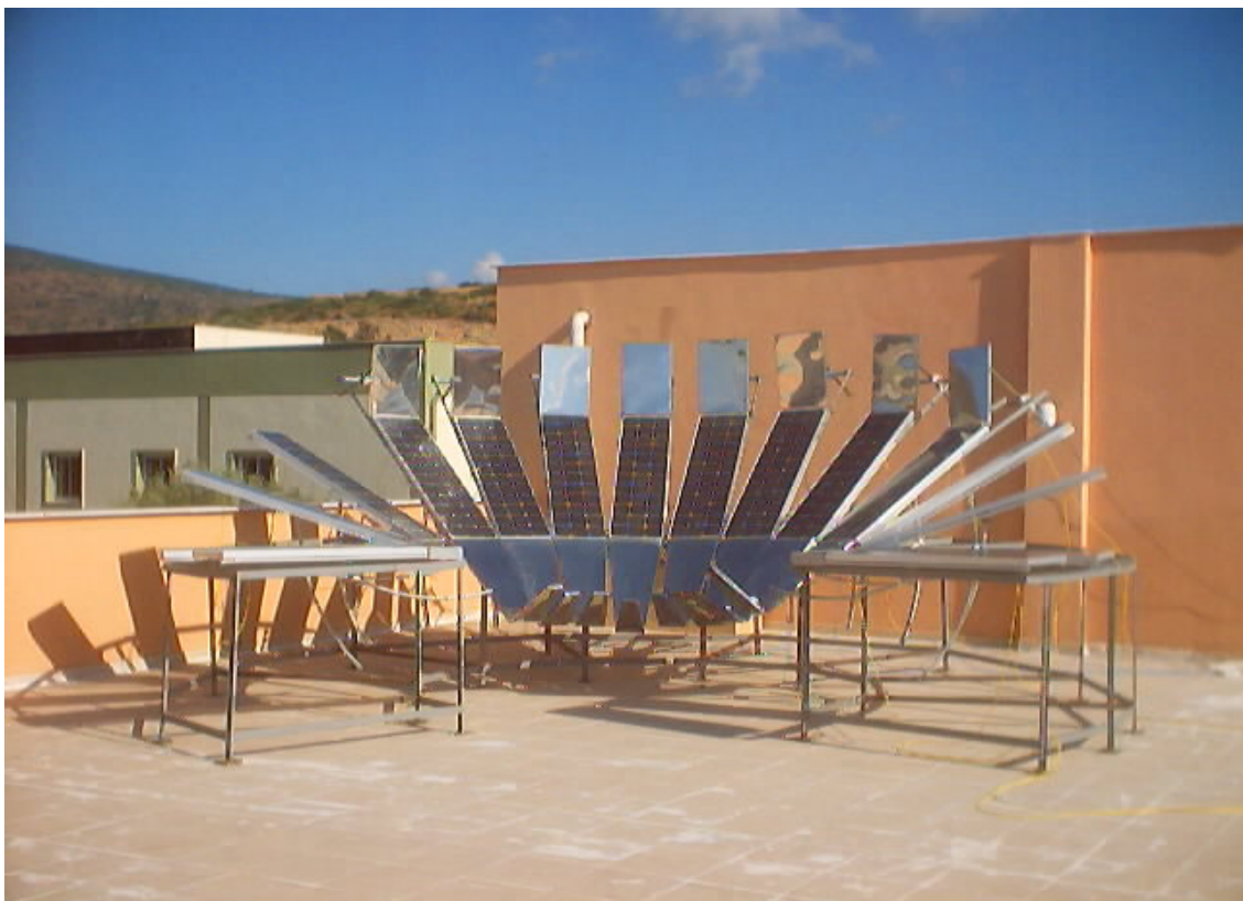
Figure 6.28 Omega Type Solar Charge Station with Optimum Inclination Angles.
