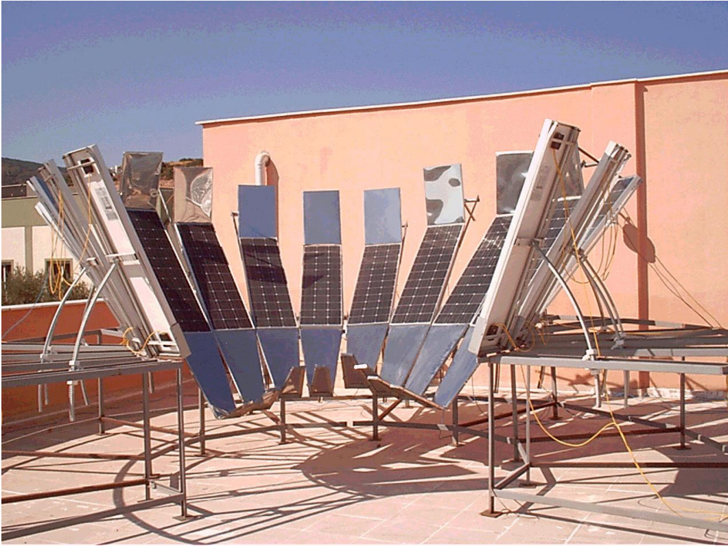
Figure 6.17 Omega Type Solar Charge Station Experiments with Reflectors.
