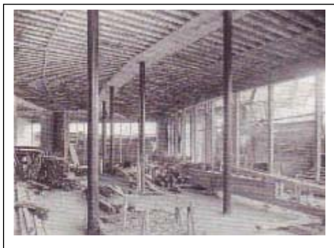
Figure 2.55. The construction of the Post Office in Goetheplatz by Robert Vorhölzer, Munich, 1931-1933
