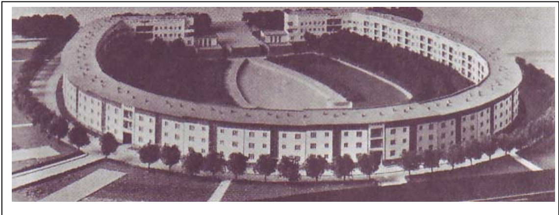
Figure 2.31. The model of the Horseshoe Housing Development by Bruno Taut, Berlin, 1925-1930 (Source: Brenne, Tomisch, Borgert & Celasun 2005: p. 93)
