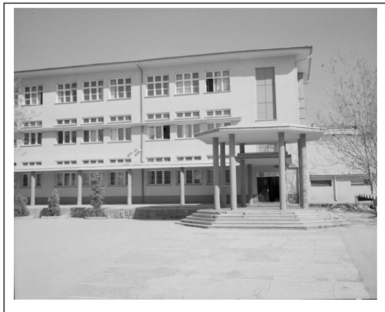
Figure 4.47. The entrance of the Atatürk High School by Bruno Taut, Ankara, 1937-1938 (Source: Photograph by Katja Eydel)
