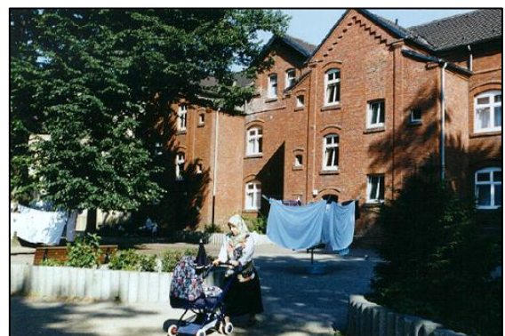
Figure 56. Worker Housing Estates 'Elisenhof' (Source: WEB_46 2006)
