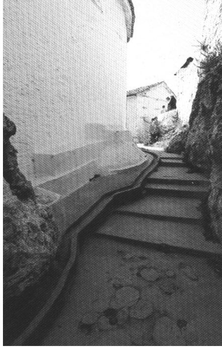
Figure 3. 21: Muğla. Drainage solution on the stairway is remarkable. (Source: Bektaş 1996)
