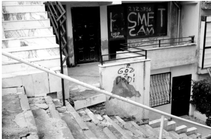
Figure 5. 81: 270 th street (September 2000)
