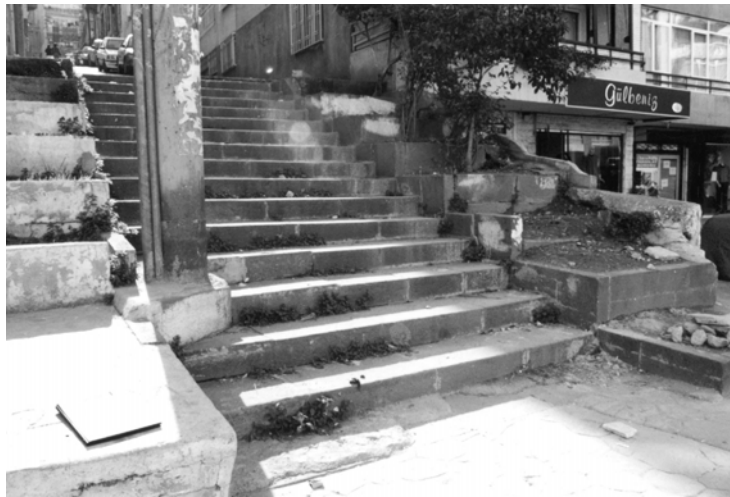
Figure 5. 28: 178 th street (September 2000)
