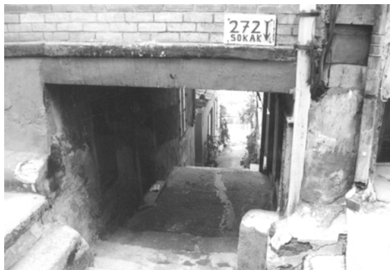
Figure 5. 40: Entrance to the covered stairway (272 nd street) from Şehit Nihat Bey Street (September 2001)
