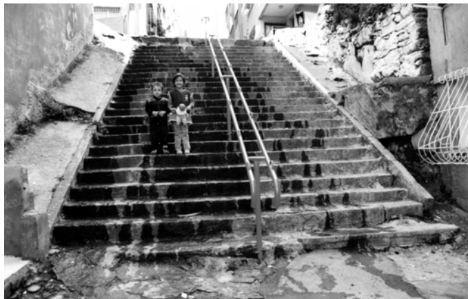
Figure 5. 74: Handrail includes a rail for each direction on 274 th street (October 2001)
