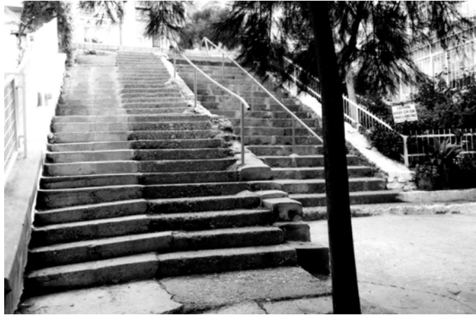
Figure 5. 72: Stairway in 111 th street has two handrails (September 2001)
