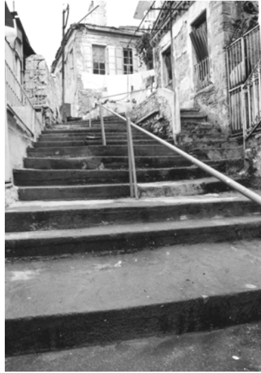
Figure 5. 38: Accent on 272 nd street to approach the covered stairway (II) (September 2001)
