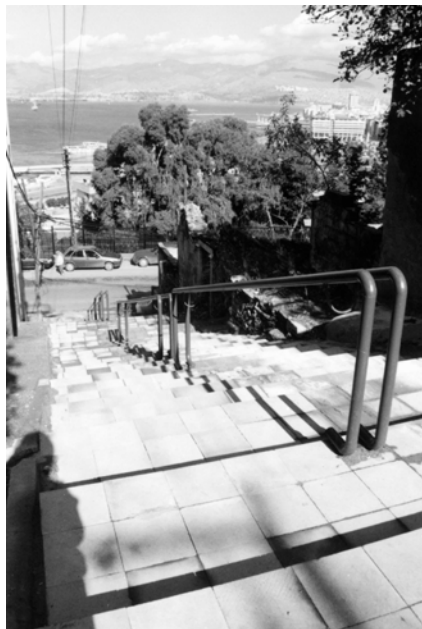
Figure 5. 73: Double rails on 402 nd street (August 2001)
