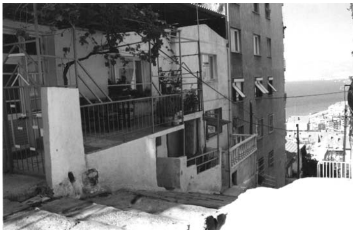
Figure 5. 83: Entrance to the building in different doors on 364 th street (August 2000)
