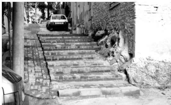
Figure 5. 53: 335 th street (September 2001)
