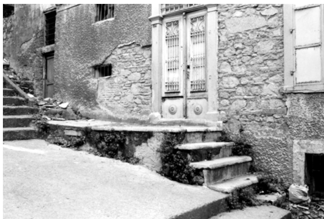
Figure 5. 92: Entrance to the building on 307 th street (October 2000)
