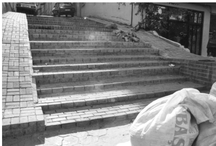
Figure 5. 29: 138 th street (October 2001)
