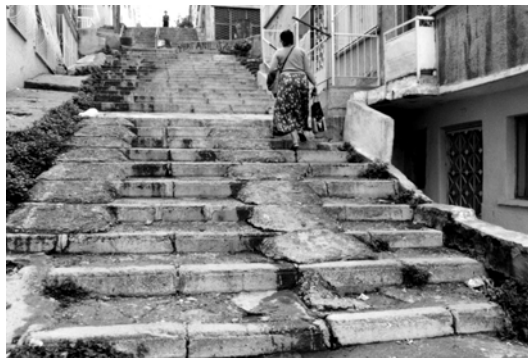
Figure 5. 55: Existing concrete steps and ramps on 271 st street (September 2001)
