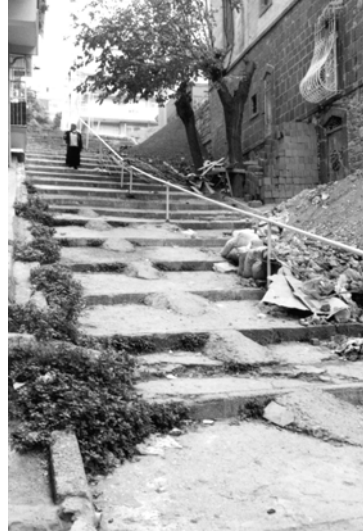
Figure 5. 54: Existing concrete ramp solution on 186 th street (September 2001)
