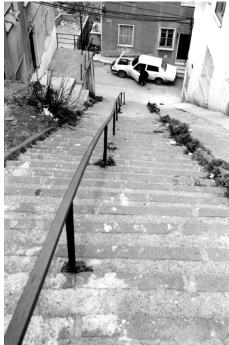
Figure 5. 45: Stairway in 314 th street without landings (September 2001)
