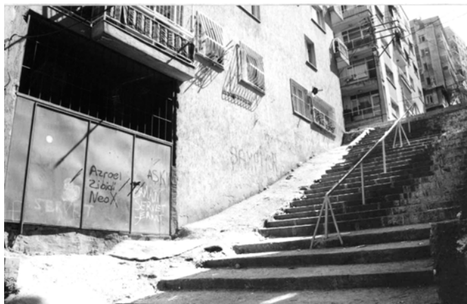
Figure 5. 98: Steep ramps obstructed with entrances (September 2000)
