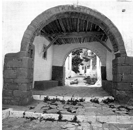
Figure 2. 17: Covered stepped passageway in the Archontoyeitionia (Philippides 1983)
