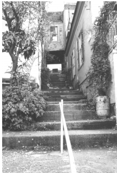
Figure 5. 39: The covered stairway on 272 nd street (September 2001)
