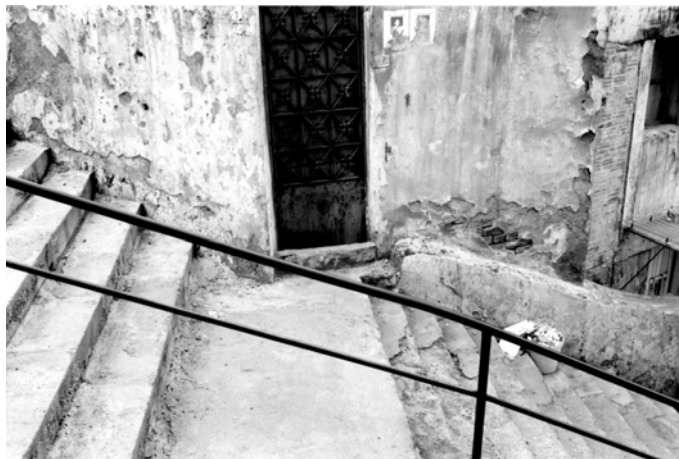
Figure 5. 97: Landing providing access to the building (September 2000)
