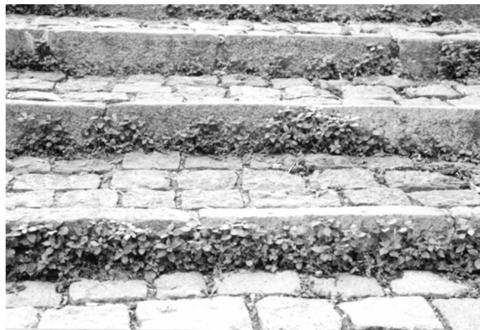
Figure 5. 60: Cobble stone pavements on 305 th street (May 2001)
