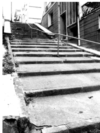
Figure 5. 59: A part of 274 th street's steps has large treads
