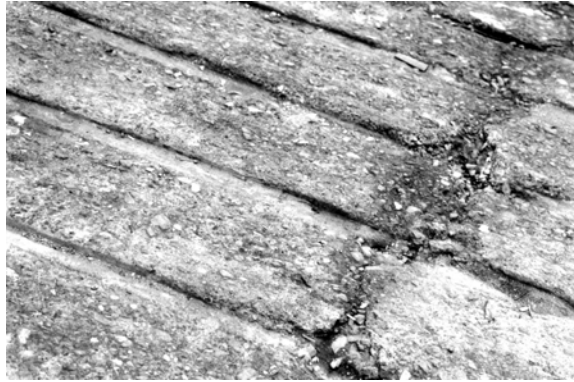
Figure 5. 57: Transforming stairway to the ramp in 282 nd street (September 2001)
