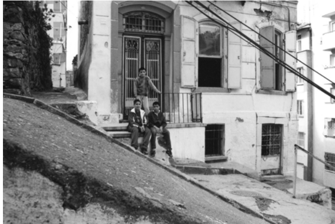
Figure 5. 84: 269 th street (October 2000)
