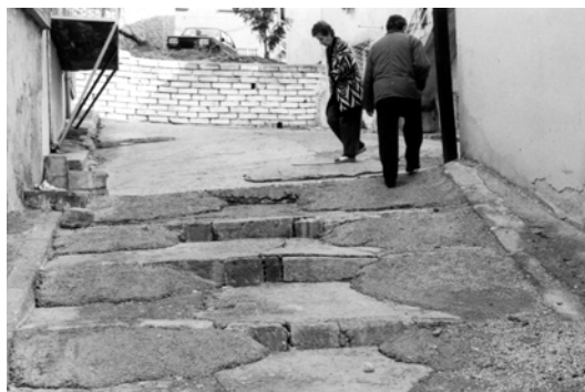
Figure 5. 56: Existing ramps on 353 rd street (September 2001)
