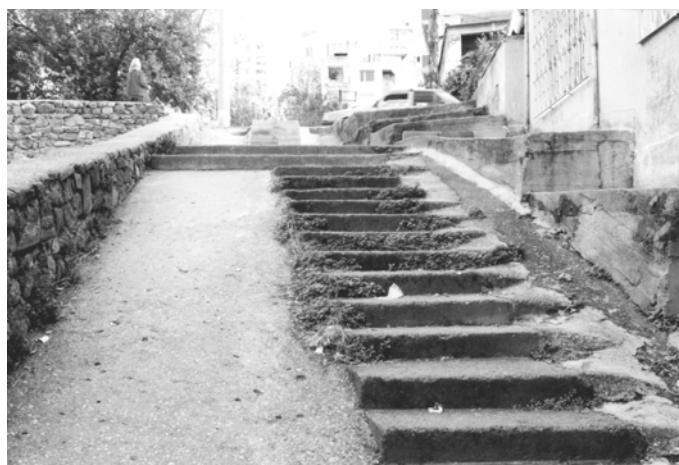
Figure 5. 50: Ramp solution along the stairway on 349 th street (August 2001)
