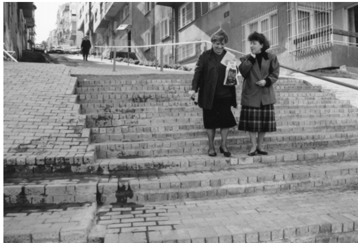
Figure 5. 25: 179 th street (October 2001)
