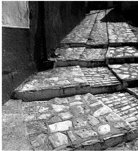
Figure 4. 24: Drainage system on stairways in Pano Vathy (Source: Philippides 1983)
