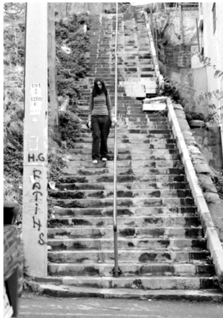
Figure 5. 46: Steep topography does not allow appropriate frequency for landings on 341 st street (September 2001)
