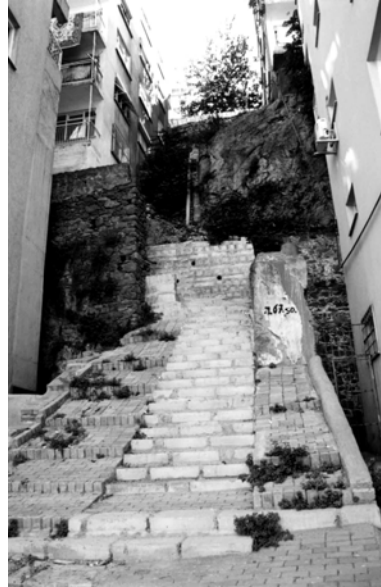
Figure 5. 19: The first flight of the stairway as connector on 167 th street (August 2001)
