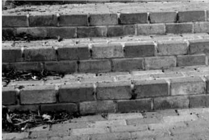
Figure 5. 65: Pocket stone steps on 100 th street (August 2001)
