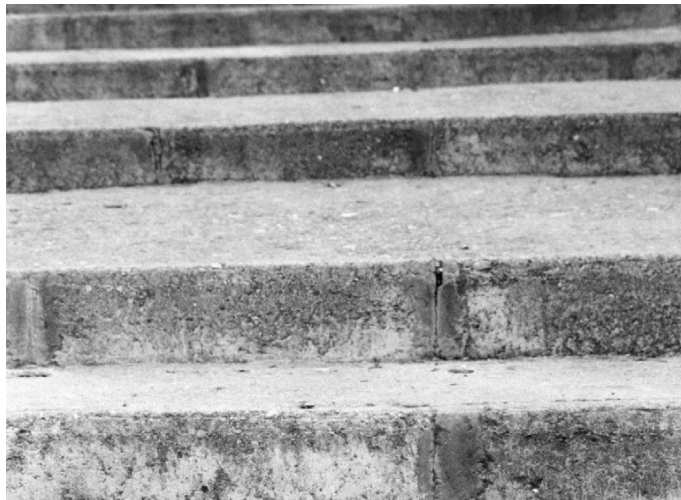
Figure 5. 63: Concrete steps on 249 th street (September 2000)
