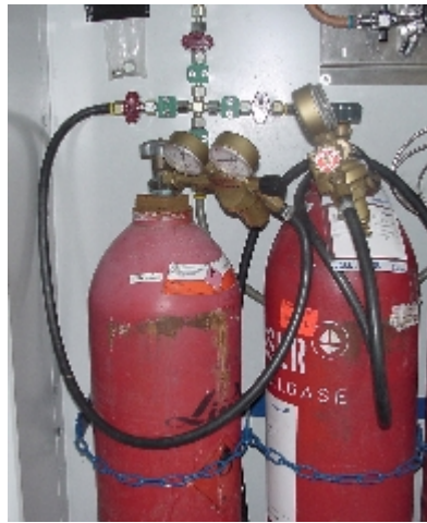
Figure 4.9. Methane gas bottle with pressure regulation valves
