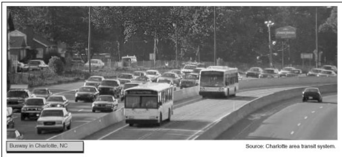
Figure 2. 13 Busway in Charlotte
