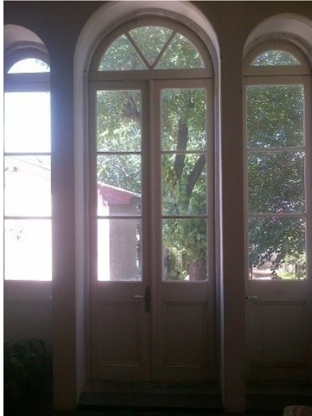
Figure 5.14. Wooden frame, arc shaped exterior doors
