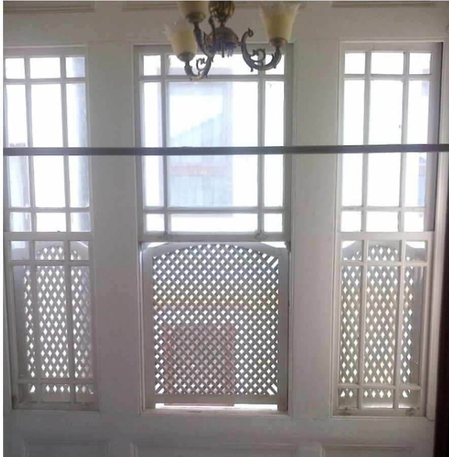
Figure 5.13. A window with wooden lattices on the cumba
