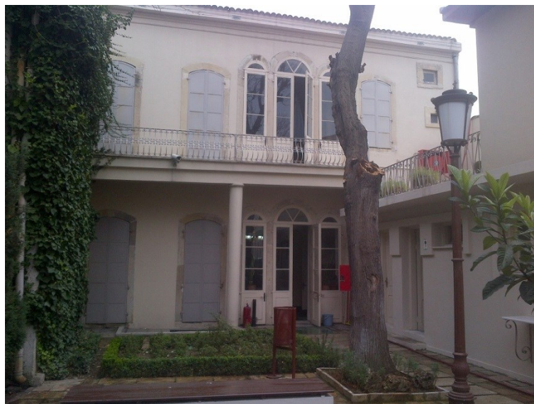
Figure 3.17. Shutters on the west façade
