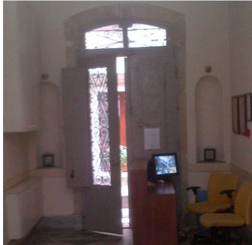
Figure 3.16. The external door
