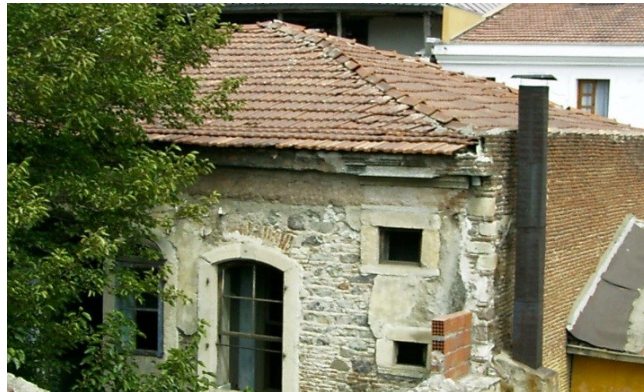
Figure 3.15. Pitched roof before restoration (Source: Dept. of Architectural Restoration - IZTECH)
