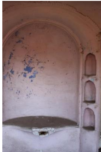
Figure 94. A view of the arced niche on closet system in F11
