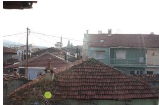
Figure 8. A view of the neighbour buildings
