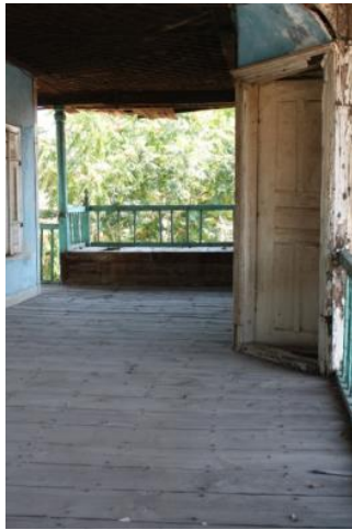
Figure 61. A view of the hall- F01, the platform to sit
