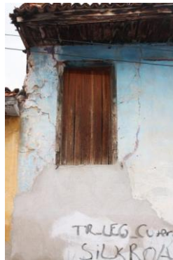
Figure 106. A view of the door (A2F3) that opens to street directly
