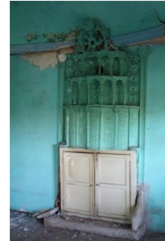
Figure 82. A view of the fireplace in F08- room
