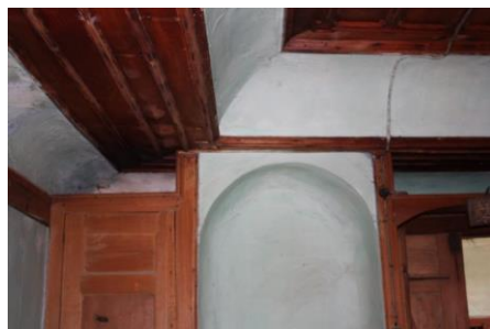
Figure 68. A view of F02- room, its ceiling and closet system
