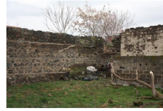
Figure 117. A view of the additional wall and debris in the garden.
