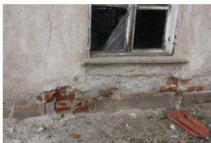
Figure 144. The southwestern wall of the G11 (room)
