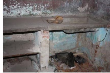
Figure 21. A view of the additional kitchen counter in B01 (kitchen)
