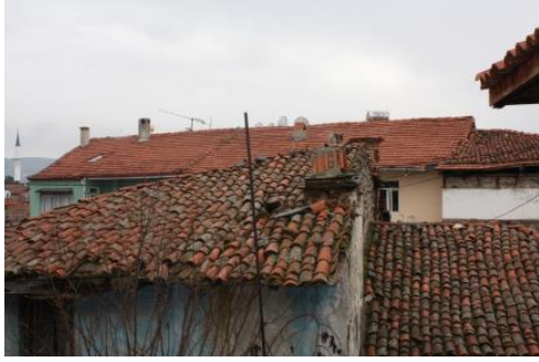
Figure 108. A view of the roofs of annex-1 and annex-2
