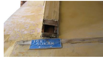
Figure 135. A view of bracket and its finishing layer
