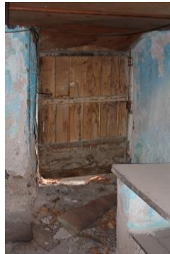
Figure 19. A view of entrance door from B01 (kitchen)
