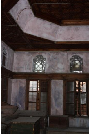
Figure 70. A view of the room- F03
