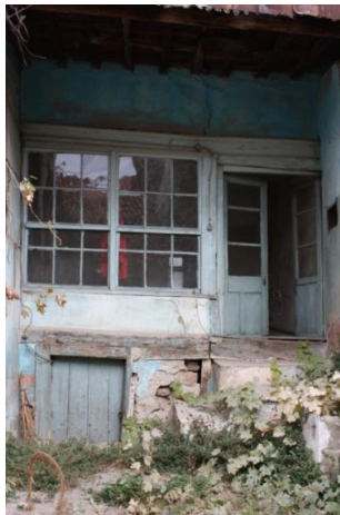
Figure 22. The courtyard entrance of B02 (hall)
