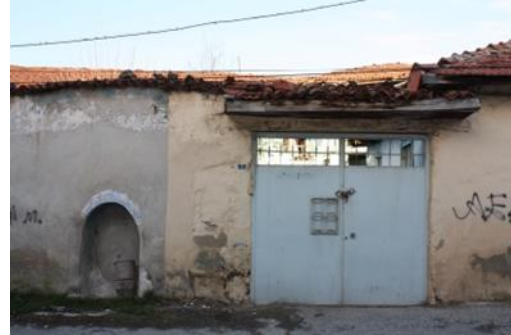
Figure 17. A view of courtyard entrance door of unit- 3
