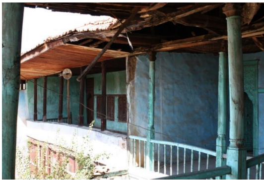
Figure 59. The addition walls that divide the hall into three parts
