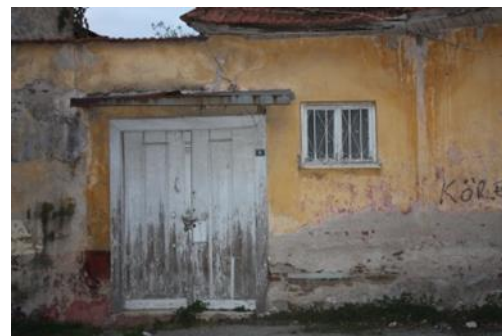
Figure 15. The courtyard entrance door of unit-1
