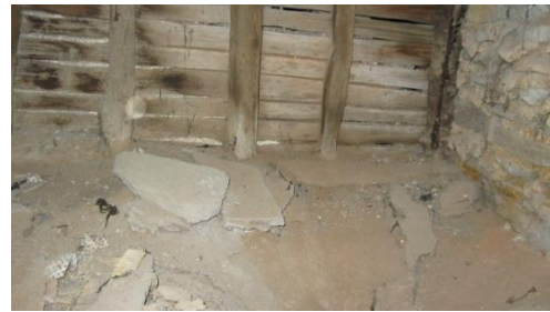
Figure 56. A view of the furnace space
