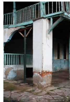
Figure 141. A view of the additional pier on courtyard facade
