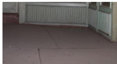
Figure 145. A view of converted floor covering
