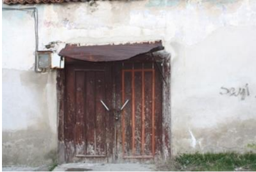
Figure 16. A view of courtyard entrance door of unit- 2
