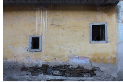
Figure 104. A view of the service space windows of annex- 1
