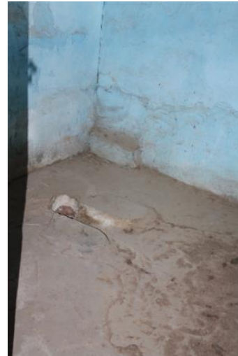
Figure 92. A view of F09- toilet
