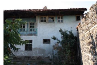
Figure 119. A view of the service space windows that open to garden
