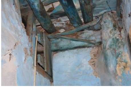
Figure 36. A view of the shutter in the toilet (B11)
