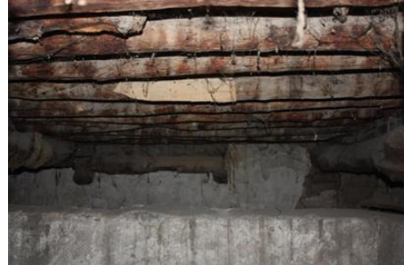
Figure 25. A view of the B03- storage from its window opening
