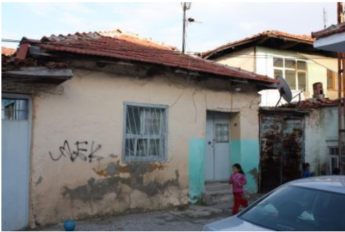
Figure 110. A view of annex-3, from the street
