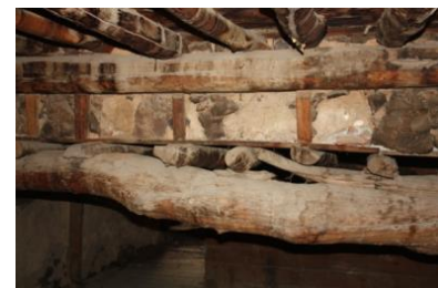
Figure 40. A view of the ceiling of the storage (B12)
