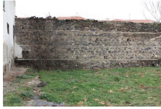
Figure 116. A view of wall of garden
