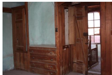
Figure 69. A view of F02- room, its floor and entrance
