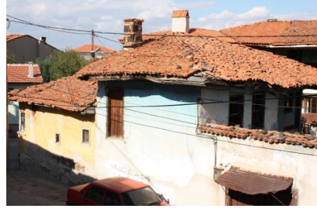
Figure 109. A view of annex-1 and annex-2 from the street
