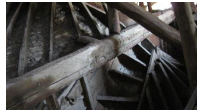
Figure 132. A view of the construction of dome and arched niche
