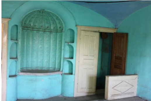
Figure 81. A view of the entrance level ( sekialtı ) and the closet system in F08- room
