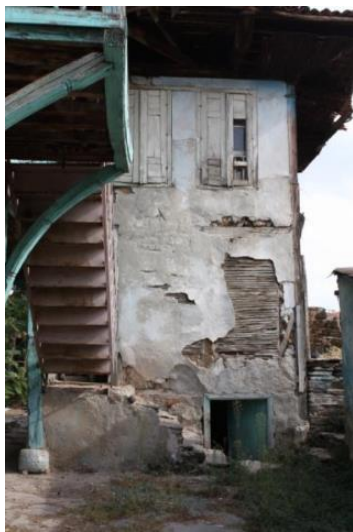
Figure 98. A view of courtyard facade
