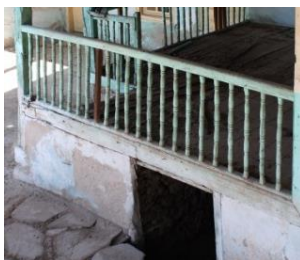
Figure 38. A view of the entrance opening of the storage (B12)
