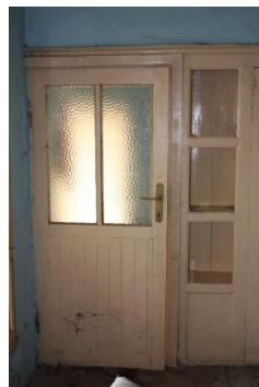
Figure 32. A view of the entrance door of B08
