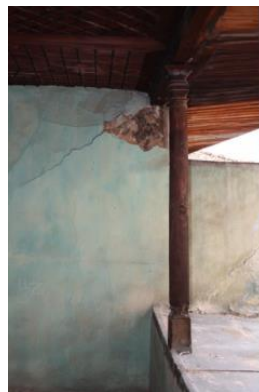
Figure 140. A view of the additional walls on the first floor
