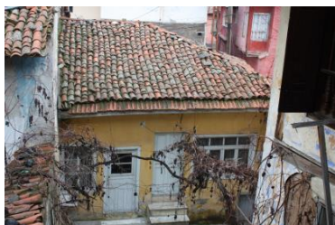
Figure 101. A view of annex- 1 from the hall (F01)
