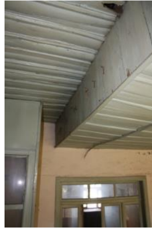
Figure 44. A view of ceiling of the hall (G01)
