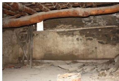
Figure 39. A view of the windows of the storage (B12)
