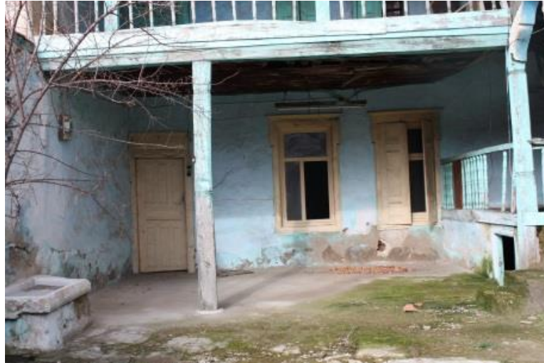
Figure 30. A view of B07- hall
