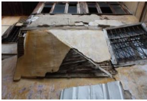
Figure 133. A view of bracket and its finishing layer
