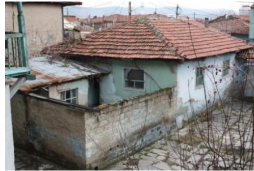
Figure 111. A view of annex-3, from the hall- F01 of Bekirbeyler House
