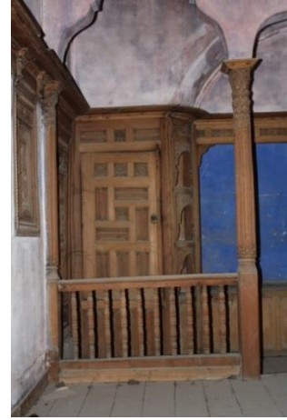
Figure 72. A view of the shutter of the gusulhane
