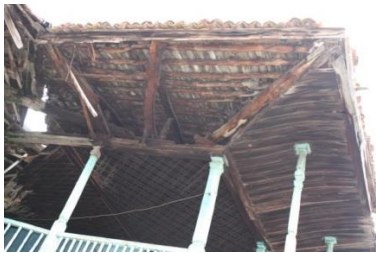
Figure 122. A view of roof and eaves
