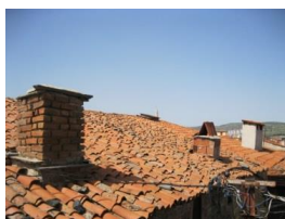
Figure 126. A view of the roof covering
