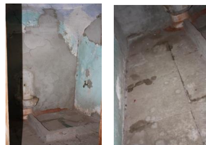
Figure 54. The views of the floor and the pendentive of flattened dome
