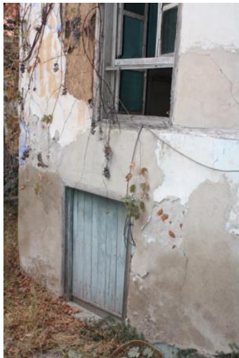
Figure 18. A view of the entrance of B01 (kitchen) from courtyard
