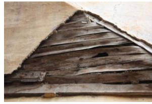
Figure 134. A view of bracket and its finishing layer
