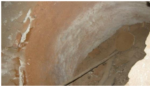
Figure 55. A view of the furnace space
