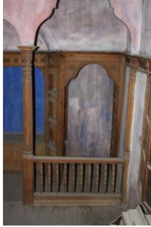
Figure 71. A view of the arcade and entrance
