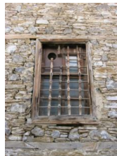
Figure 131. A view of the rear facade wall
