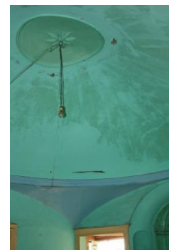
Figure 84. A view of the dome and pendentives
