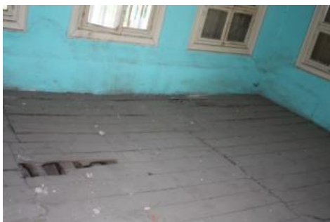
Figure 45. A view of floor of G02-room
