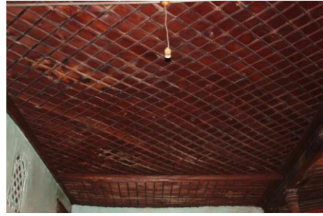
Figure 67. A view of the ceiling of F01- hall
