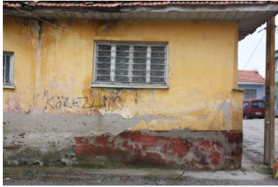
Figure 103. A view of annex- 1 from 168 street
