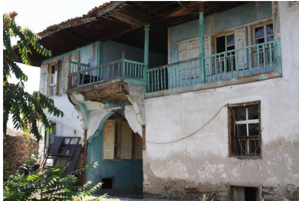
Figure 96. A view of the southeastern (garden) facade
