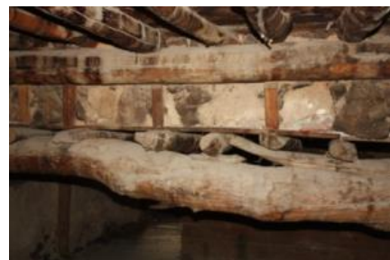
Figure 52. A view of floor system of the hall (G09)
