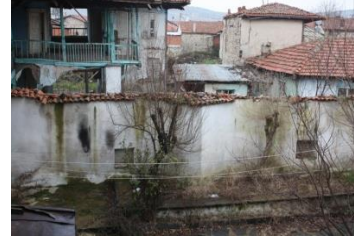
Figure 113. A view of addition wall in the courtyard
