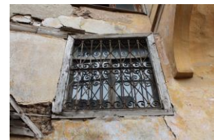
Figure 146. Additional iron grill
