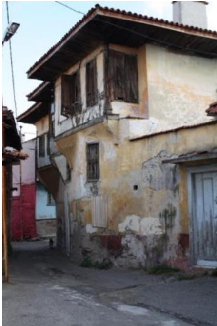
Figure 2. A view of the Bekirbeyler House from the 168 street
