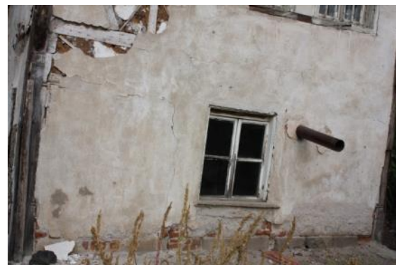
Figure 58. A view of the renewed wall of the room- G11
