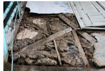
Figure 125. A view of wooden post and beam framing system
