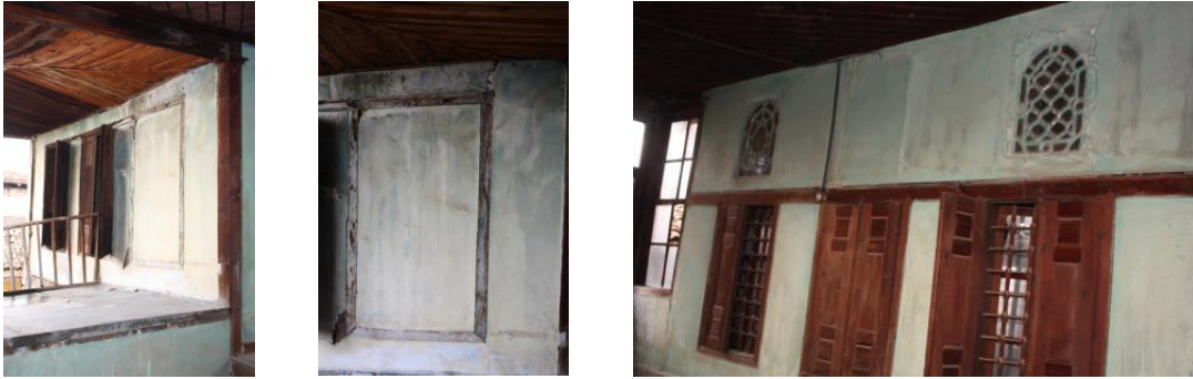
Figure 147. Missing elements, closed windows in the main building a) F02 (room) b) frame of the window c) closed top window in F01 (hall)
