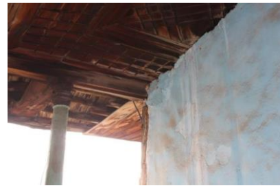
Figure 138. A view of the additional walls on the first floor
