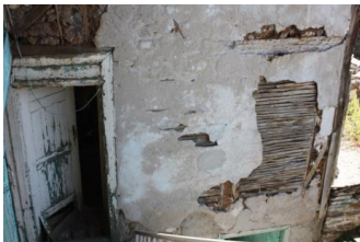
Figure 130. A view of the finishing with the technique of wooden lath
