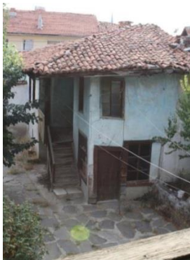
Figure 105. A view of annex- 2 from F01
