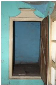
Figure 85. The shutter in F08- room
