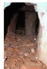
Figure 90. A view of the duct which extends under the gusulhane
