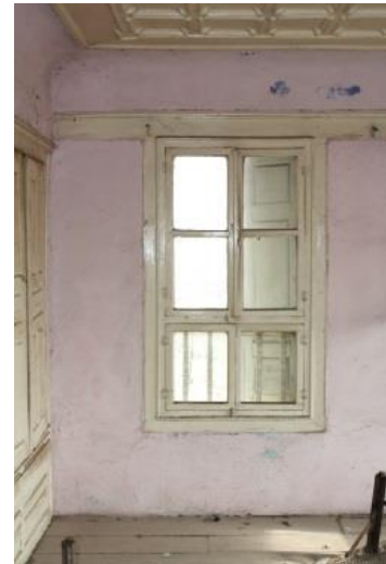
Figure 95. A view of the window, floor and ceiling of F11
