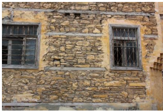
Figure 124. A view of the stone masonry wall
