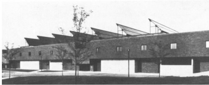
Fig.3.55. Solar energy collectors on the roof of St. George's School (Source: Gordon et al., 1990, p.319)
