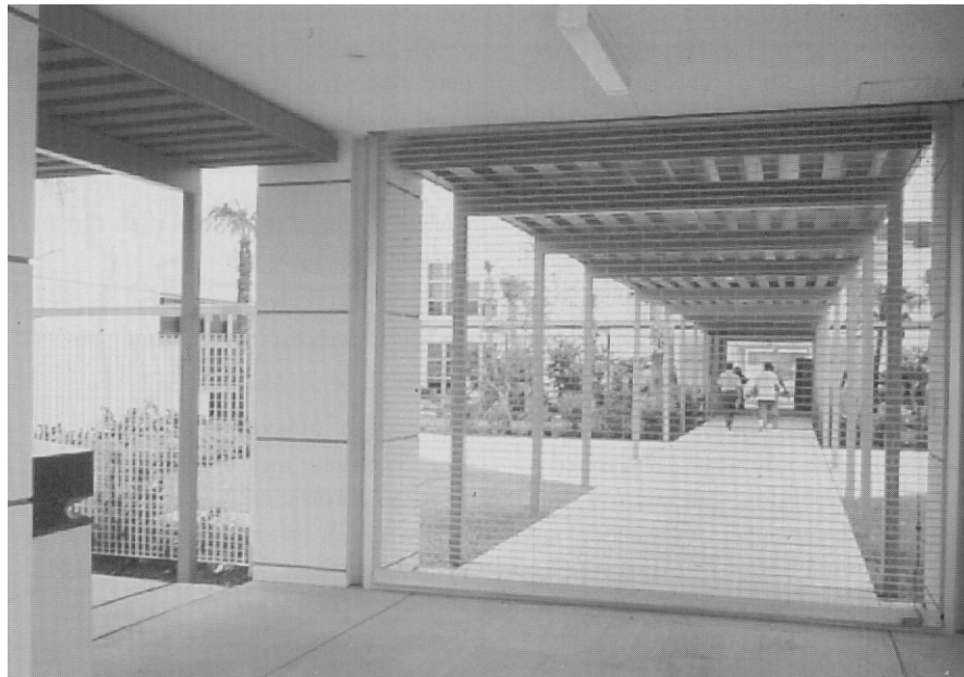
Fig.3.7. Middle school prototype, Broward County Florida: As transparent security element, grills are used between indoor and outdoor circulation paths. If the grills are removed the school is open. (Source: Perkins, 2001, p.190)
