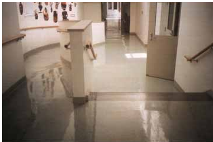
Fig.3.20. Ramp and stairs should be designed together. Handicapped students need to interact and not be discriminated. (Source: Karabey, 1998, p.83)
