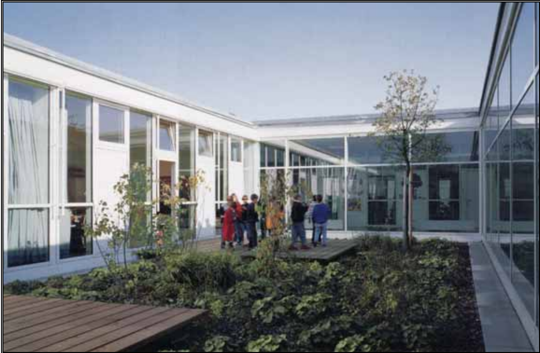
Fig.3.17. Primary School in Vienna- Each classroom has its own garden. The school structure is formed by succession of small courtyards which also enables surveillance.
