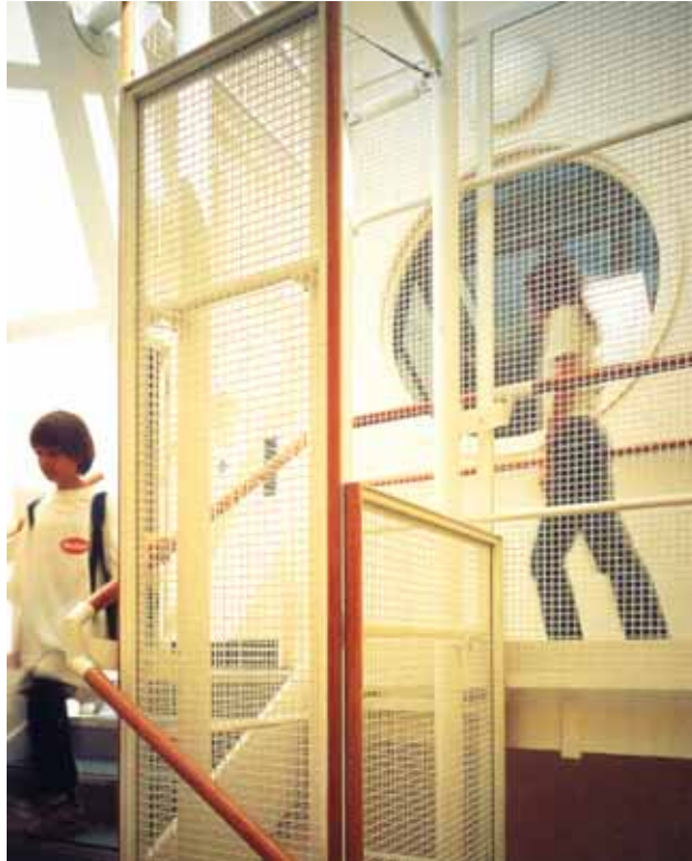
Fig.3.5. Security precautions of stairwell along handrails in Fairley House School Pimlico, London, UK (Source: Jestico + Whilo, Educational Spaces , 1998, p.14)
