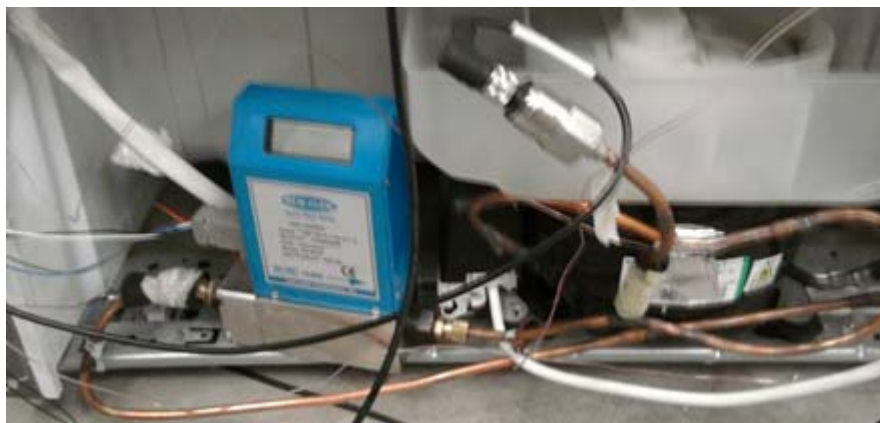
Figure 3.11. The mass flow meter connection at the inlet of the compressor
