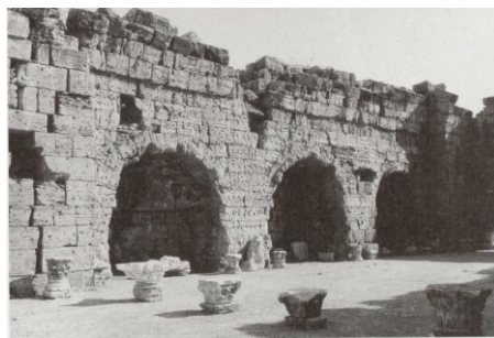
Figure 2.28. Stone northern wall of the caldarium of Hierapolis Bath (Source: Yegül, 2011)
