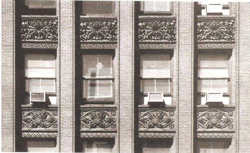
Figure 45. A Detail of the Facade of the Wainwright Building (Source: Elia, Louis Henry Sullivan , 79.)
