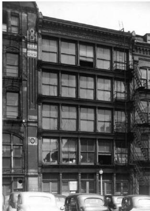
Figure 5. A View of the Thomas Gantt Building (Source: Historic Architecture and Landscape Image Collection, Ryerson and Burnham Archives, The Art Institute of Chicago, Reproduction, in Murray, Contemporary Curtain Wall Architecture , 17.)
