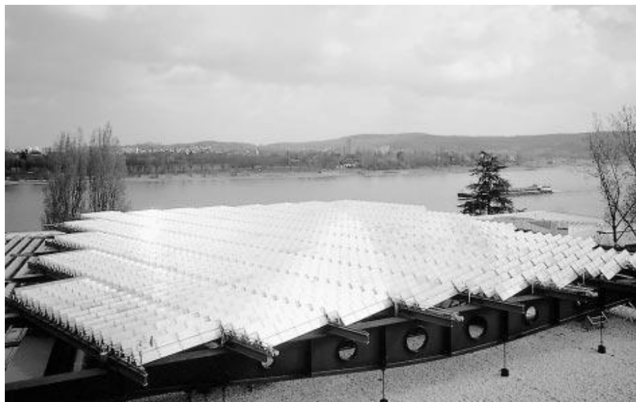
Figure 2.10. Prismatic panels - German Parliament Building, Bonn (Source: International Energy Agency, 2000)
