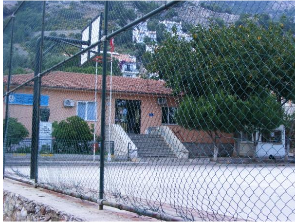
Figure 35. The building for preschool to 5 graders in Turunç
