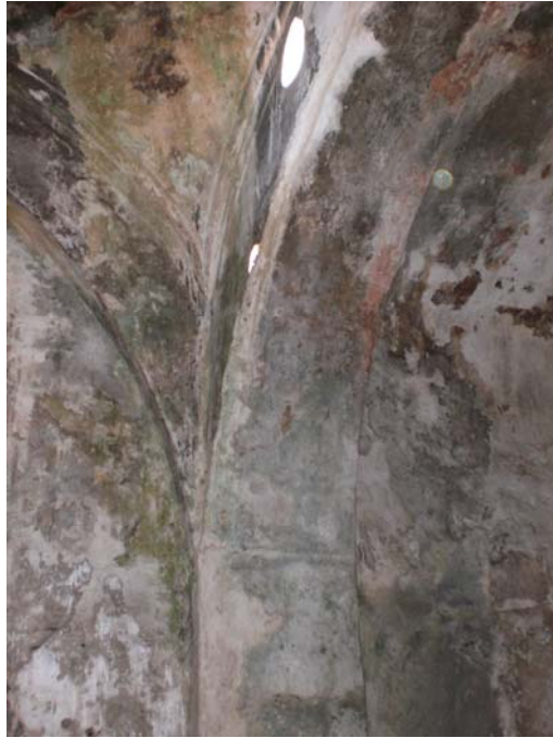
Figure 13. The pendentive encircled with border in the caldarium
