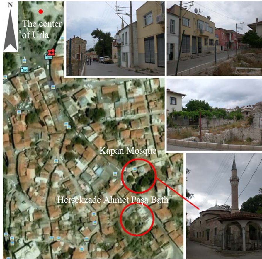
Figure 6. The satellite view and the neighboring buildings
