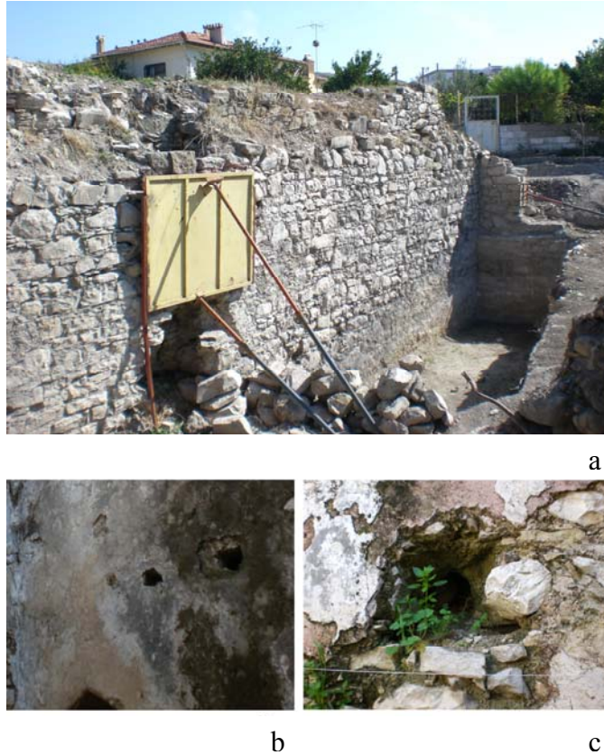
Figure 15. The southwestern exterior wall (a), the hollows on the walls in the caldarium of the men's section (b) and the wall and the brick-lime plaster on the wall in a private chamber of the men's section (c)
