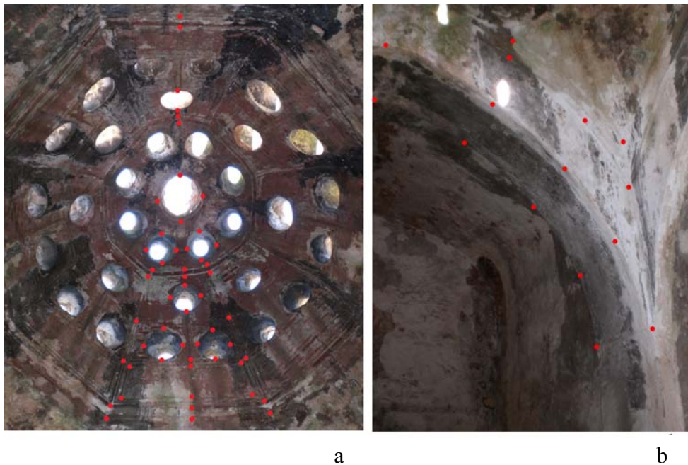
Figure 24. The points measured on the dome (a) and on an arch (b)
