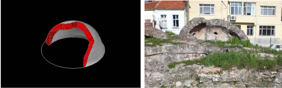
Figure 56. A partially demolished dome
