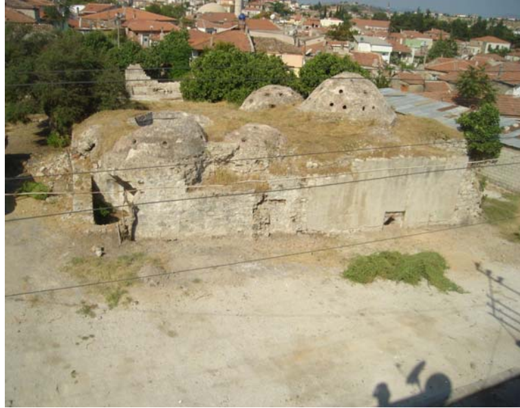
Figure 18. The eastern view of the Bath before the excavation (Source: Anka Architects 2009)
