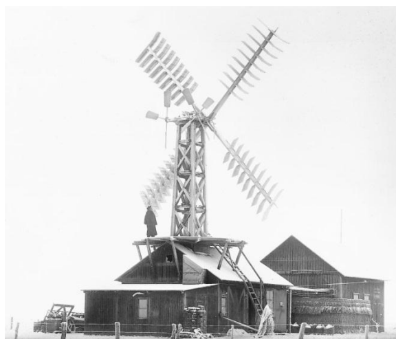
Figure 1.2. Poul La Cour's first electricity producing wind turbine [2]
