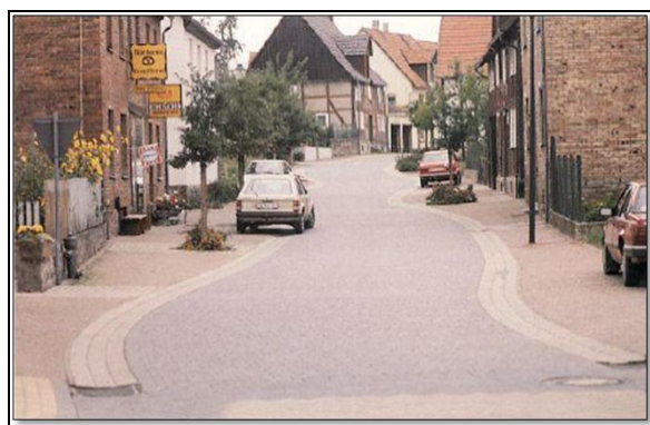
Figure 3.23. Informal side strips can enhance the appearance of village streets. Here the strips are in sympathy with the informal arrangement of buildings and side accessways. Borgentreich, Germany (Source: Devon County Council Engineering and Planning Department of 1991)
