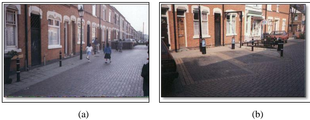
Figure 3.35.(a) Shared surface showing street furniture and coloured pavers. (b) Parking bays defined with dark brown pavers and cast iron bollards. Railings also add interest to the street scene outside a local shop. (Source: Devon County Council Engineering and Planning Department of 1991)
