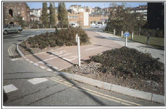
Figure 3.21. The use of red slurry seal clearly defines this section of the Exe Cycle Route (Source: Devon County Council Engineering and Planning Department of 1991)
