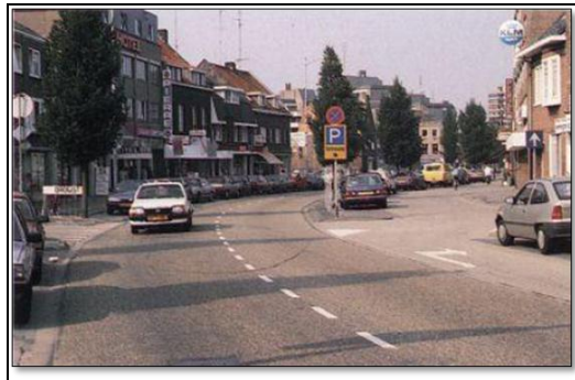
Figure 3.42. The kerb line of the original 16m wide carriageway is just visible. Within this space can now be seen a narrow carriageway, separate service road, linear parking, extended footways at corners and trees planted to soften the scene (Source: Devon County Council Engineering and Planning Department of 1991).
