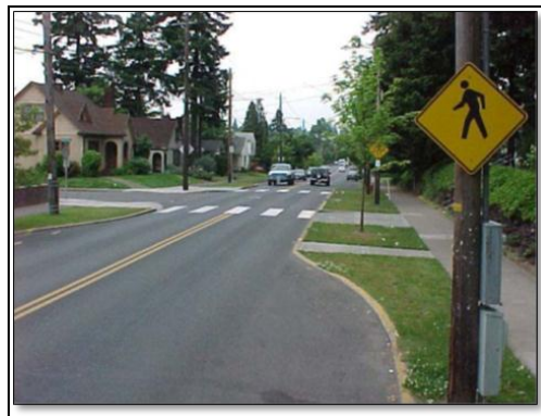
Figure 3.17 Curb extension (Source: Murphy 2003)
