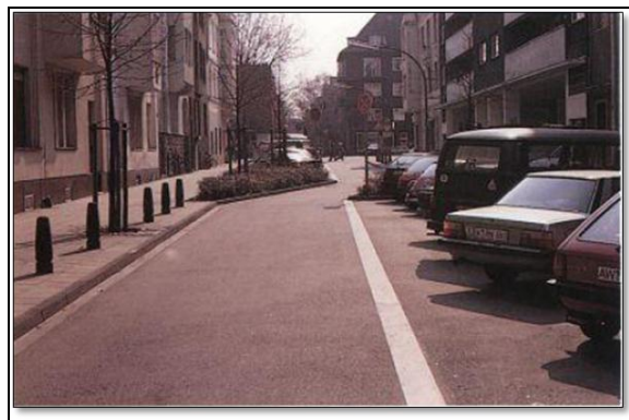
Figure 3.30. For a good speed reduction effect, lateral shifts need to be at least the width of a traffic lane, as shown here. The shift is created by the provision of alternate angled parking bays, defined by permanent planted areas. Bollards prevent parking on the footway (Source: Devon County Council Engineering and Planning Department of 1991).
