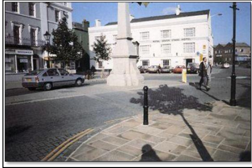
Figure 3.48. The Wills Memorial Island. The paving and footway widening has helped to reduce vehicle speeds and provided a safer and pleasanter area for pedestrians (Source: Devon County Council Engineering and Planning Department of 1991).
