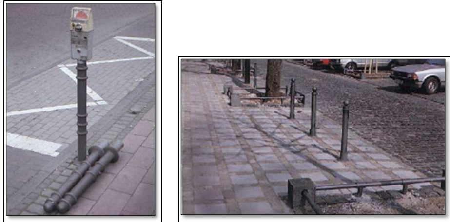
Figure 3.26. Bollards can be removable to provide access, and can serve as meter posts. Cologne, Germany (Source: Devon County Council Engineering and Planning Department of 1991)
