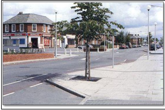
Figure 3.32. Flat top humps, lateral shifts and footway extensions at approach to junction. Planting, including raised red brick flower beds, adds to the street scene (Source: Devon County Council Engineering and Planning Department of 1991).
