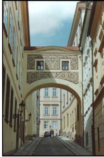
Figure 3.4: Street Arch in Prague
