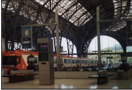
Figure 3.18: Railway Station, Barcelona.
