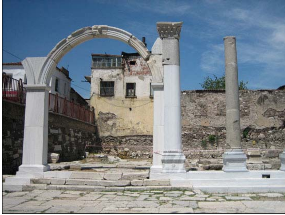
Figure 4.46. Reconstruction implementation of the West Gate and the 30 th column of the West Soa.
