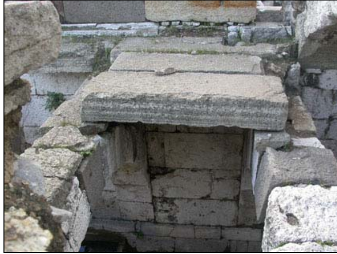
Figure 3.22. Flooring system bearing on the arches.
