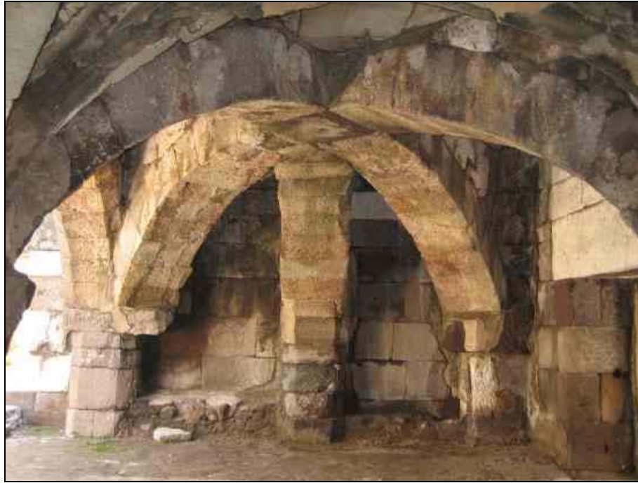
Figure 3.19. Crossed arches placed south west corner of the Basilica.
