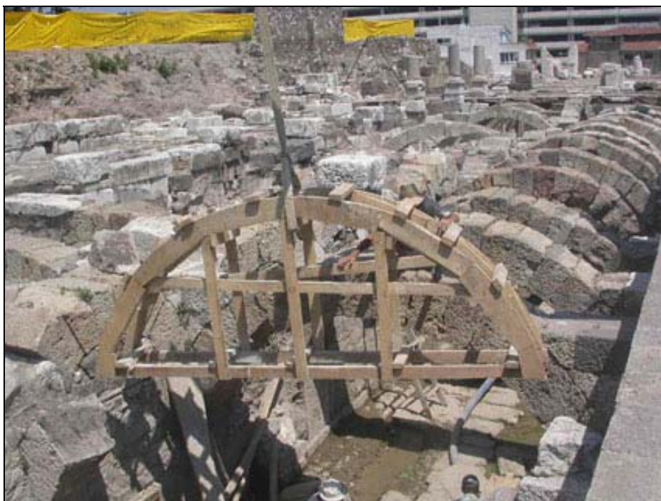
Figure 4.41. The timber staging is placed initially. (Source: Archives of the Agora excavations, 2005)
