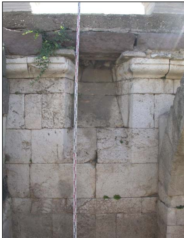
Figure 3.52. The most complete part of the wall showing the window and the mouldings.
