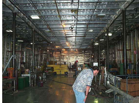
Figure 3.21. Superstructure (Source: WEB_2 2004)
