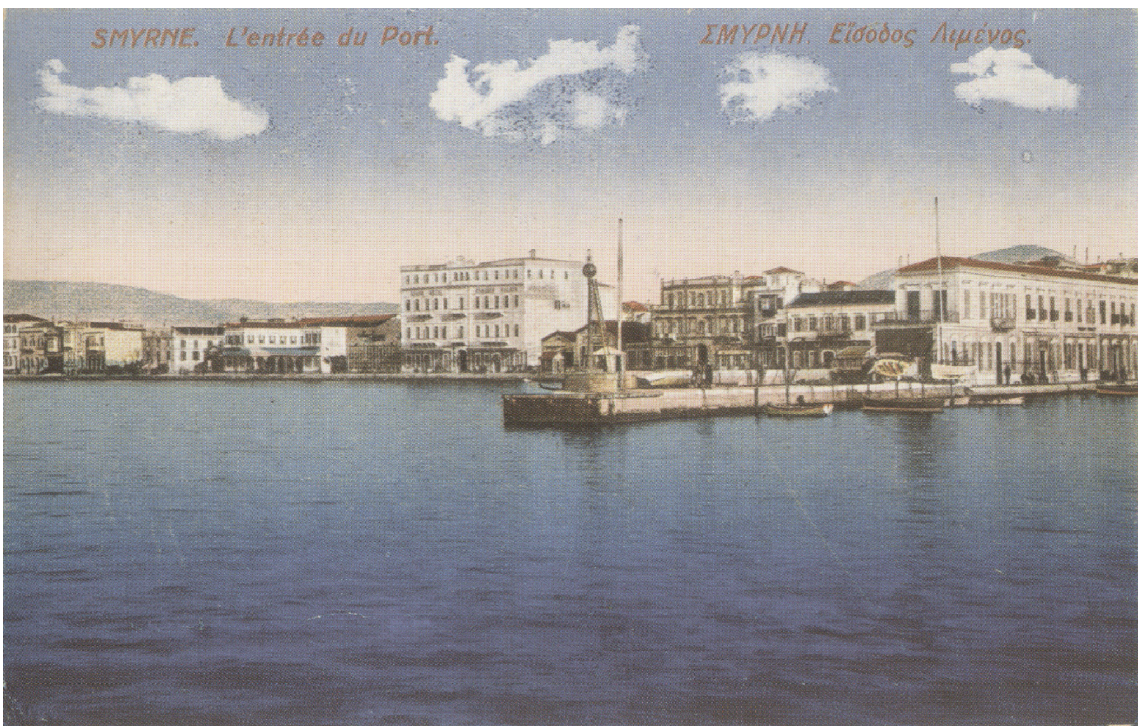
Figure 1.7. Pasaport Quay entrance (Source: Yılmaz, F. and Yetkin, S. 2003)
