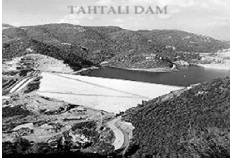
Figure C.1. General View Of Tahtalı Dam
