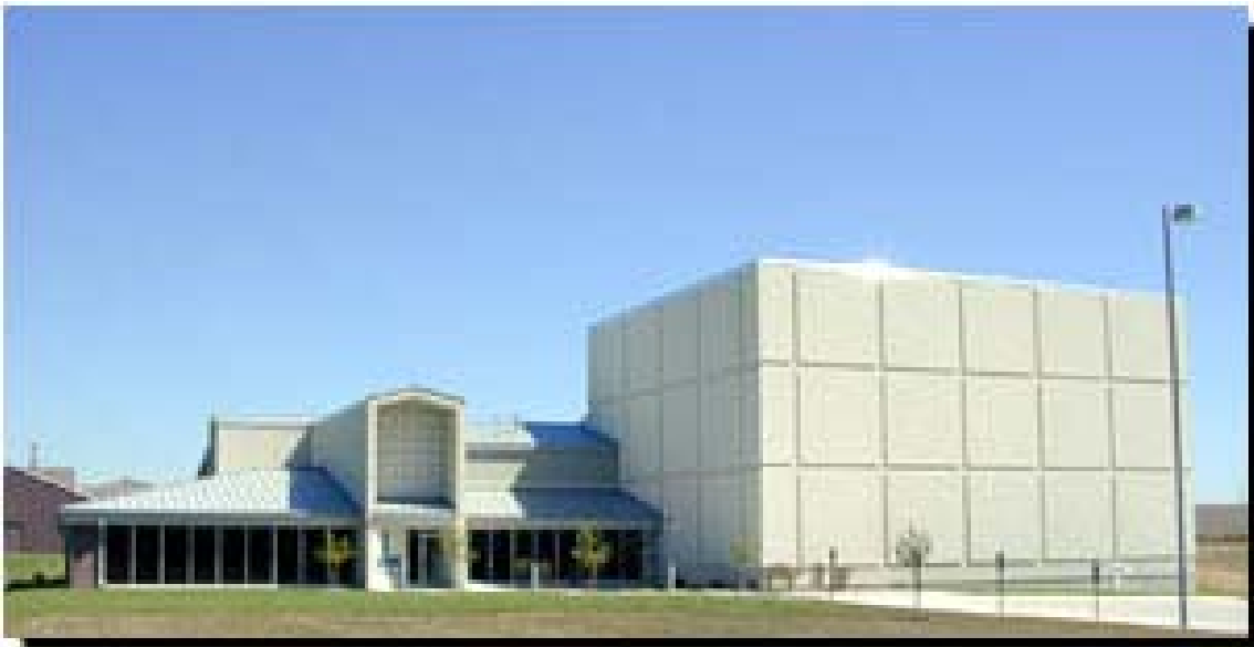
Figure D.25 The Nebraska Center (a Multitech Building)
