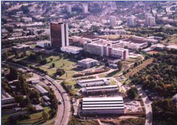
Figure D.15 Completed Zone B Production Facilities
