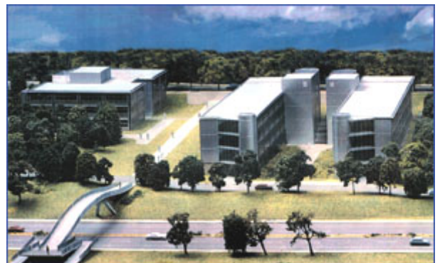
Figure D.14 Flexible accommodation totaling 28 380 m 2 suitable for office, research, technological development and production
