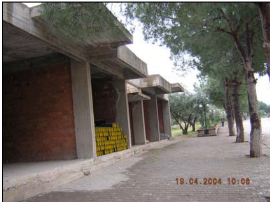
Figure A. 6 Illegal Constructions of the Municipality in 1997
