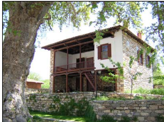
Figure A. 7 Old Geyre House near Museum
