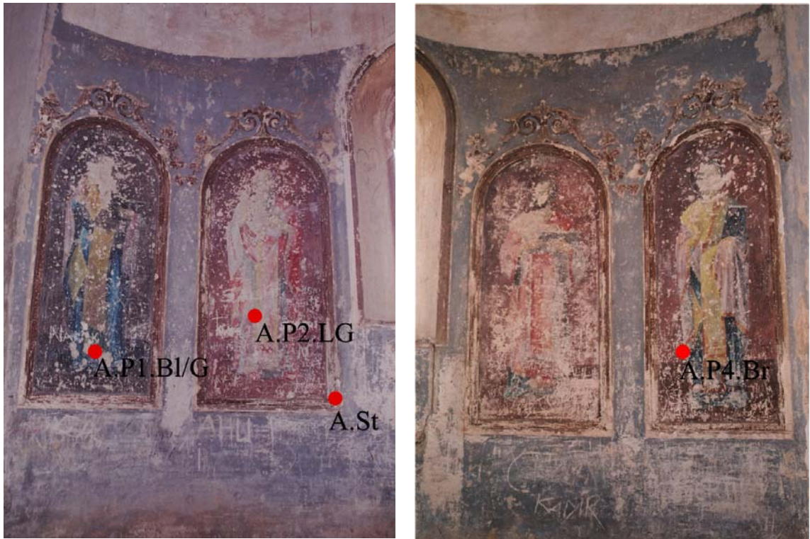
Figure 4.3. Painted plaster samples taken from the main Apse
