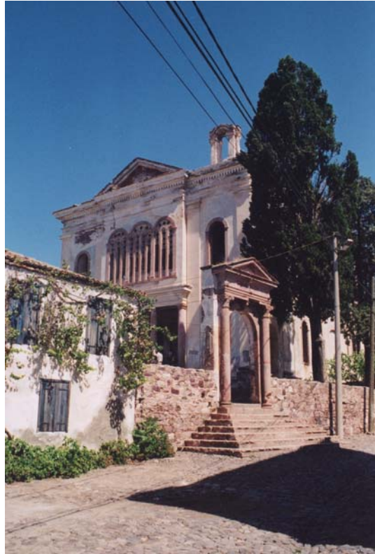
Figure 3.2. West Elevation of the Church
