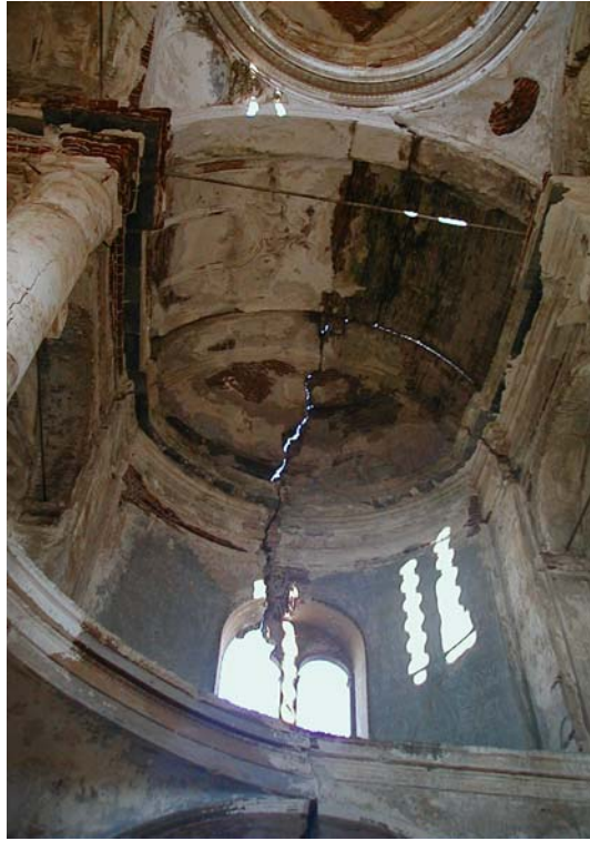
Figure 3.5. Interior view of the Church
