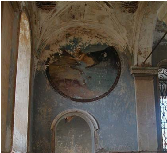
Figure 3.9. Painting over the doorway on the South of the narthex
