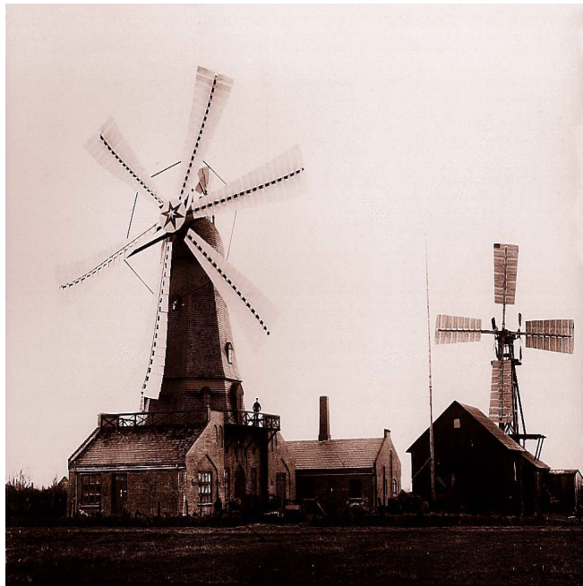
Figure 3.3. Two of LaCour's test wind turbines in 1897 at Askov Folk High School, Askov, Denmark (Source: WEB_6 2005).
