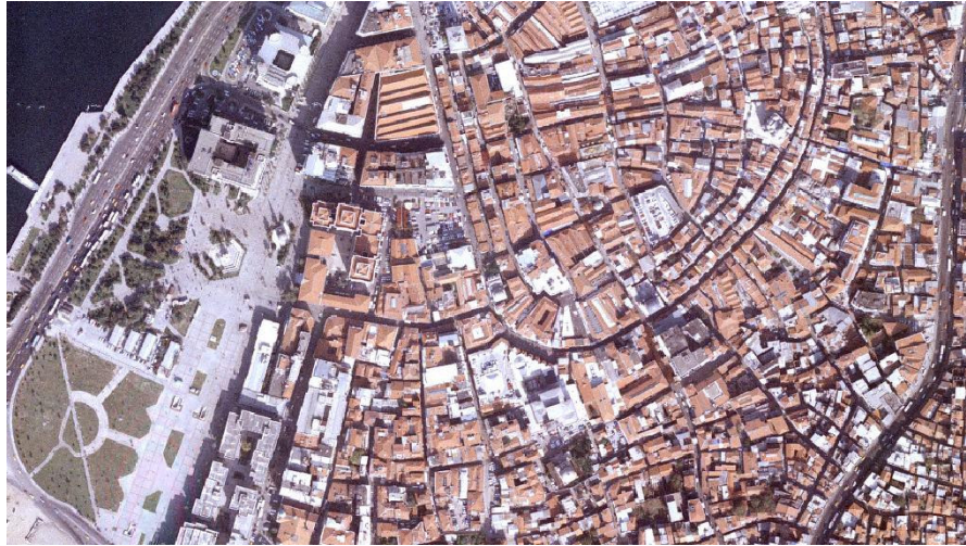
Figure 2.8. Historic Urban Fabric: Konak: Kemeraltı (Source: Izmir Metropolitan Municipality, air photo 2002)
