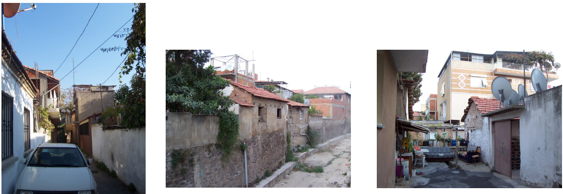
Figure 5.17. Buildings on River Bed
