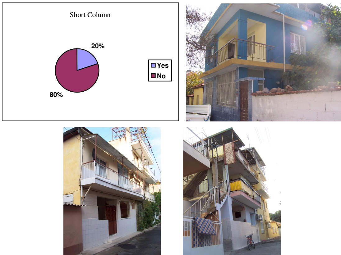
Figure 5.22. Short Column Effect
